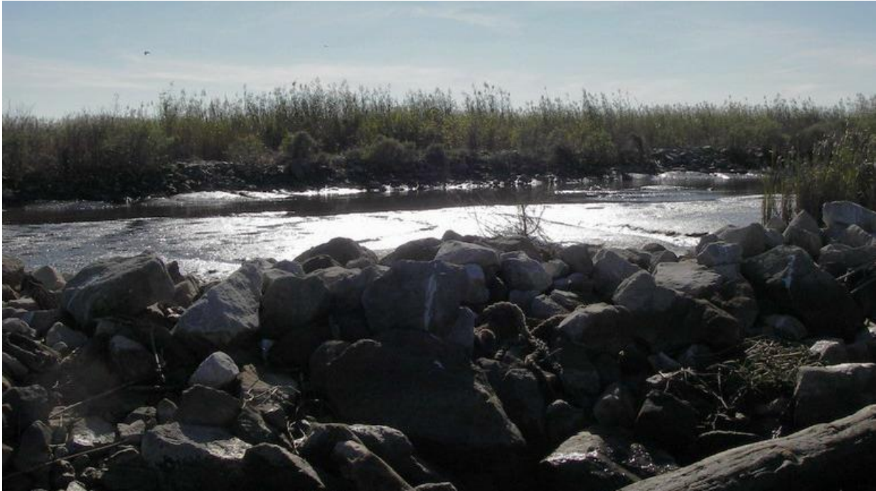
Figure 11. Sedimentation and vegetative growth between the GIWW rock dike and dredge material levee along the north side of the impoundment.
