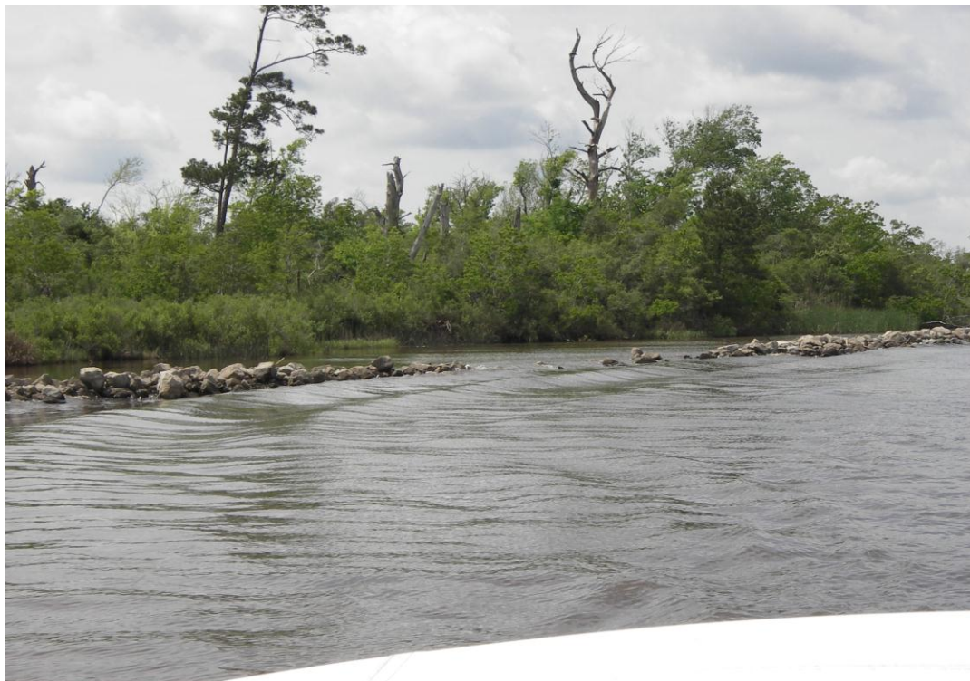
Photo 10 —Low Area of Dike Displaced by Barge
