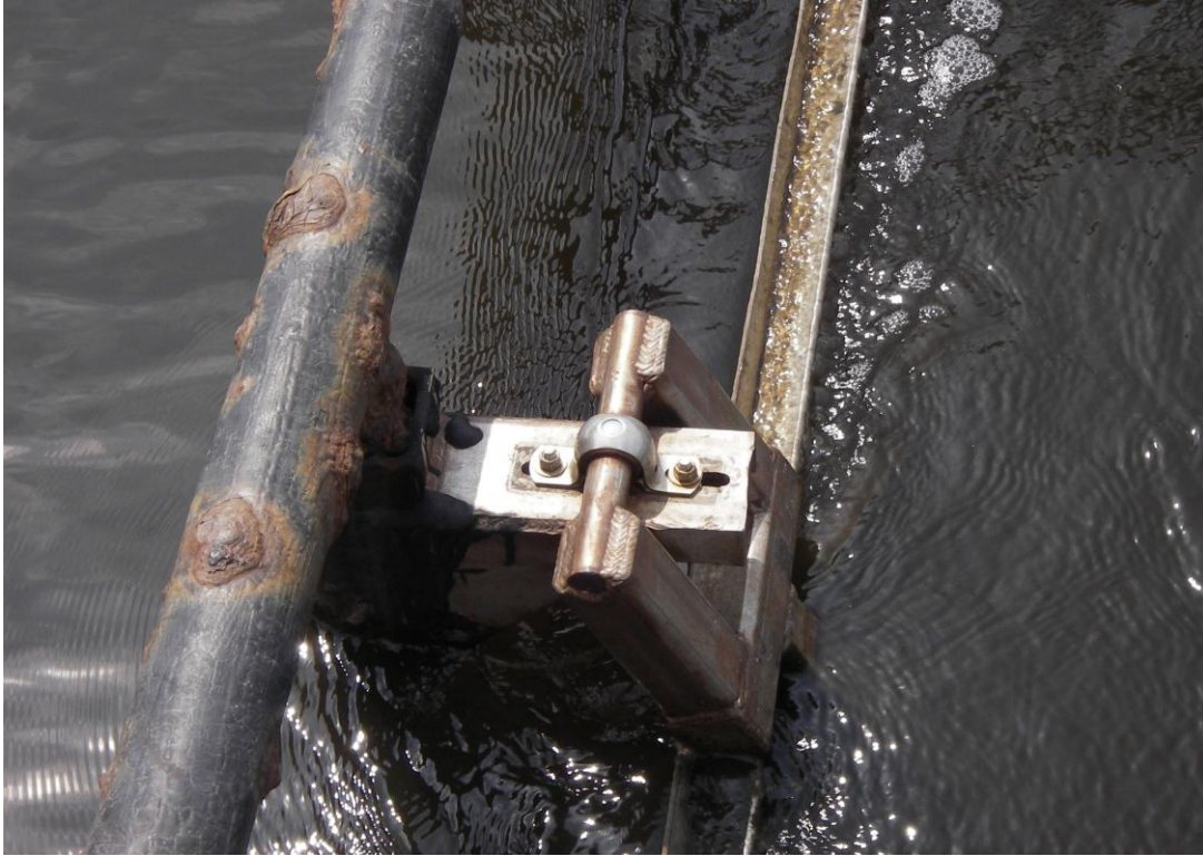
Photo 5—Pillow Block on SRT Gate Flap & Railing Rust
