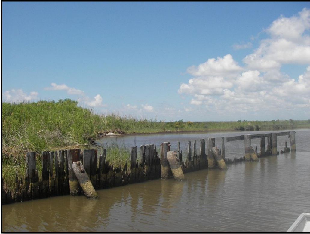
Photo 1: Area 1- Timber Bulkhead
