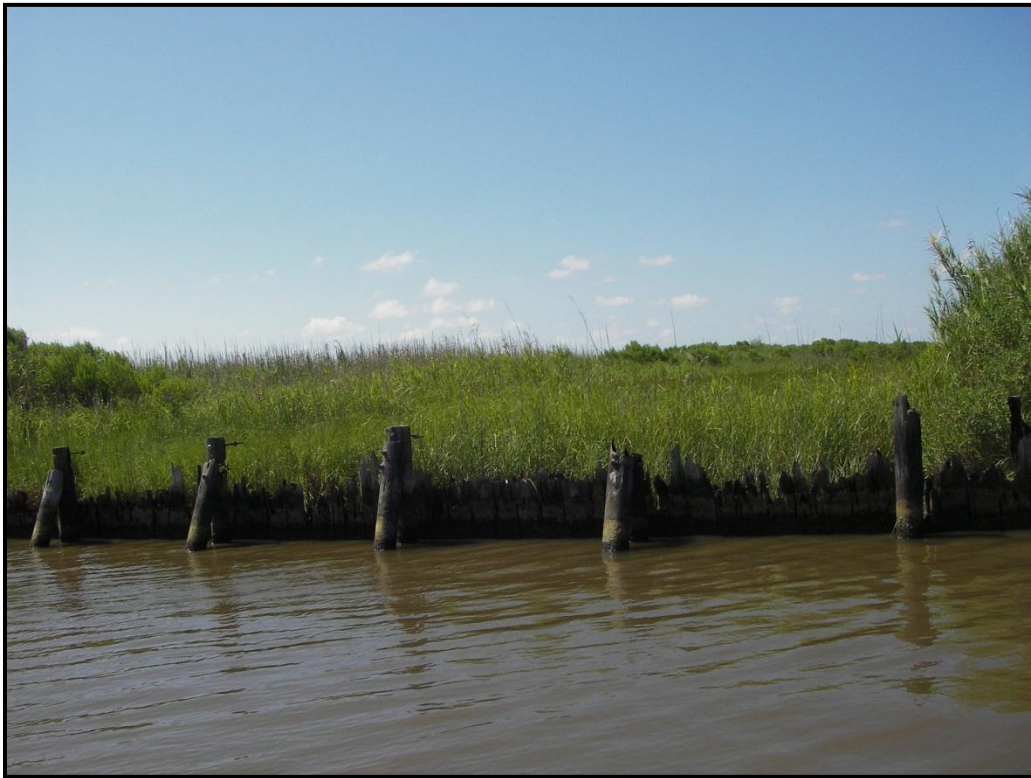
Photo 5: Area 3- Near Bulkhead on North End
