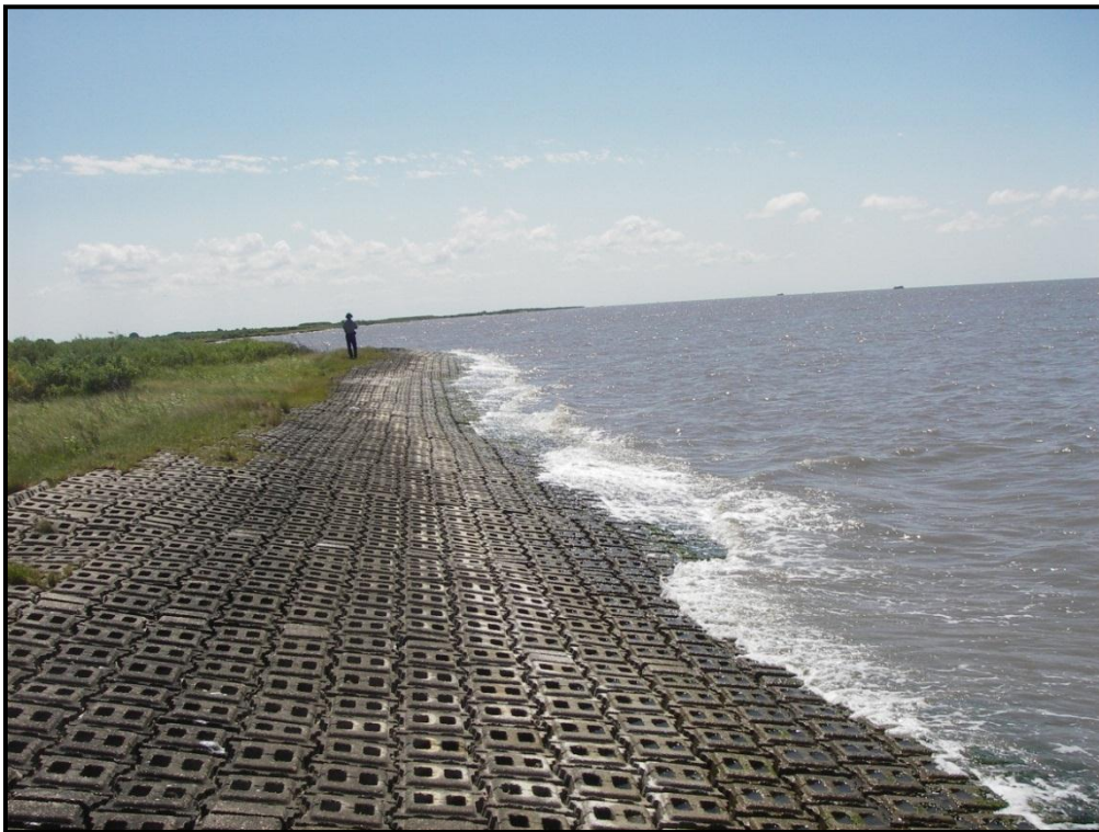
Photo 4: Area 2- East Side of Concrete Mats
