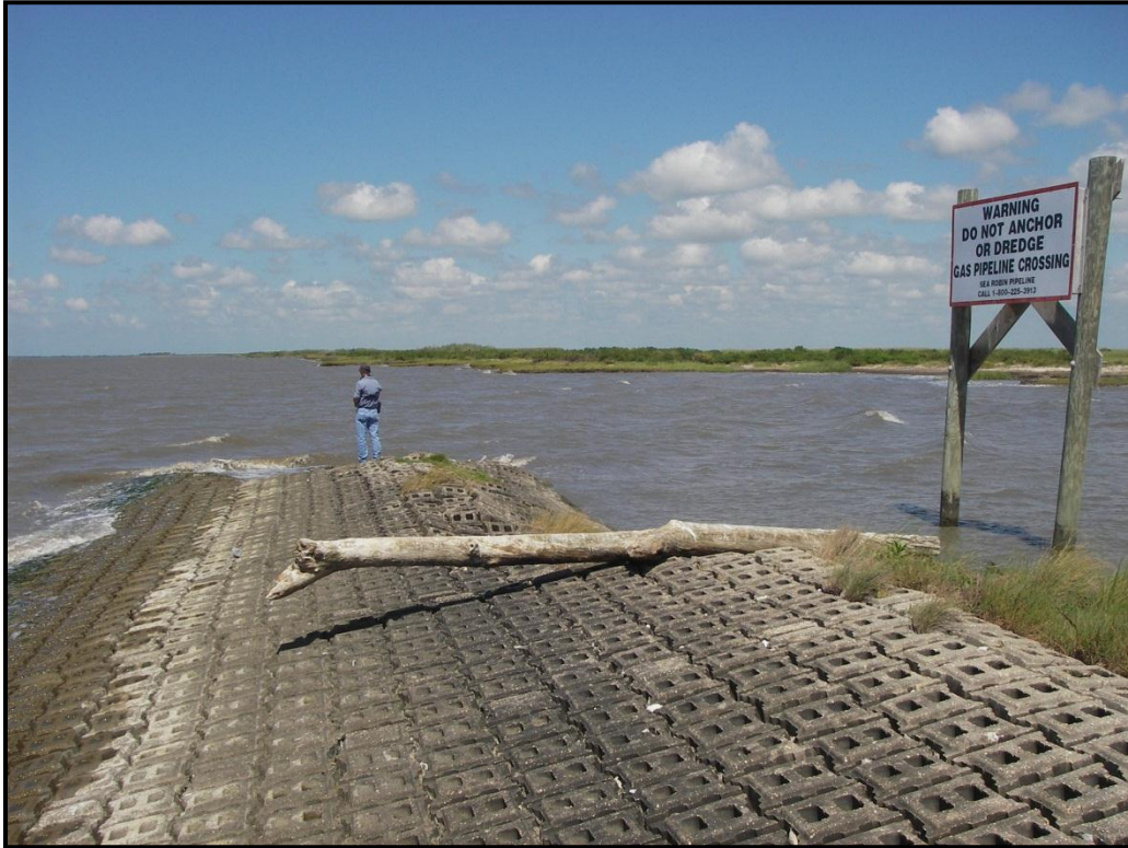
Photo 2: Area 2- West Side of Concrete Mats
