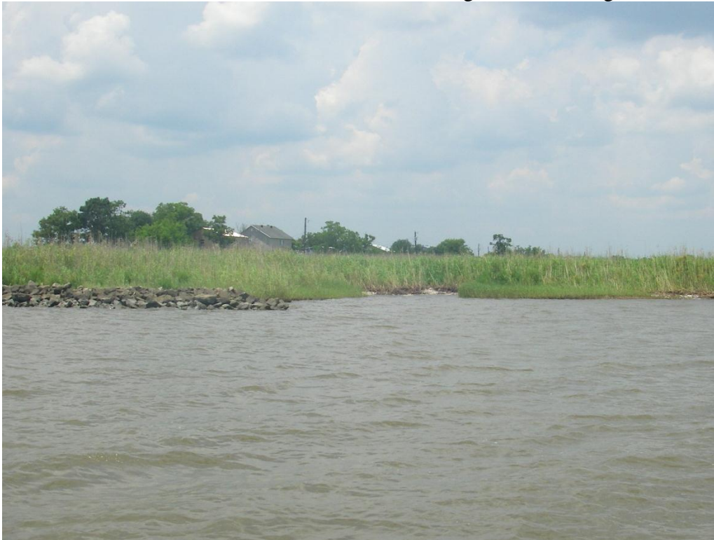
Photo No. 4, East Tie In at Shoreline
