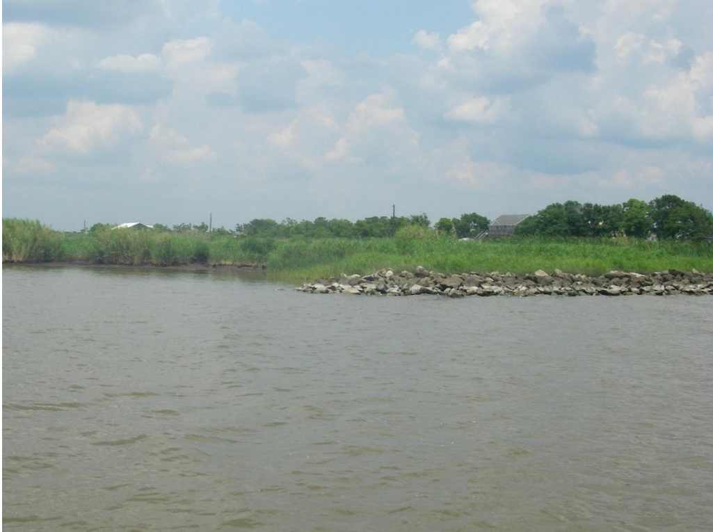
Photo No. 5, West Tie In at Shoreline
