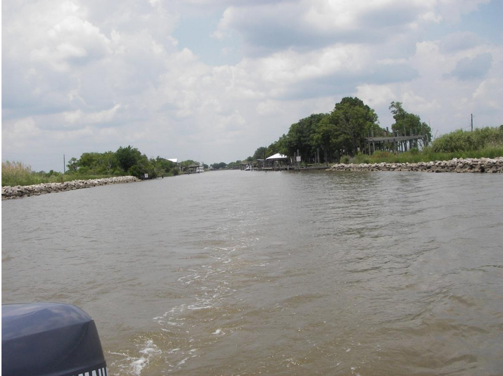
Photo No. 1, View of Boston Canal Looking North into Canal
