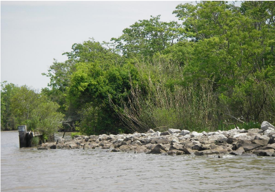
Photo No. 2 —north end of dike
