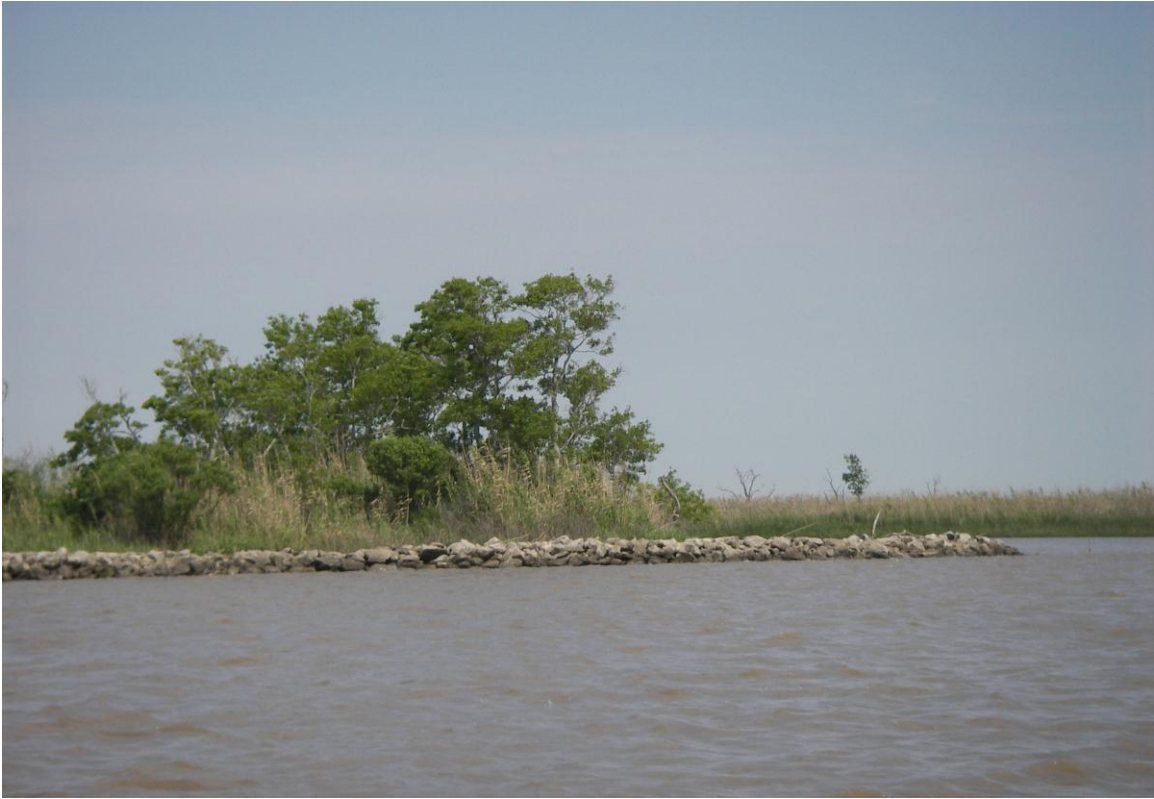
Photo No. 1 —south end of dike
