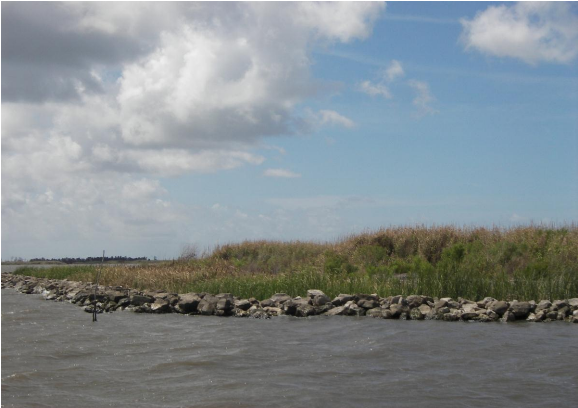
Photo No. 1 , typical section of rock dike
