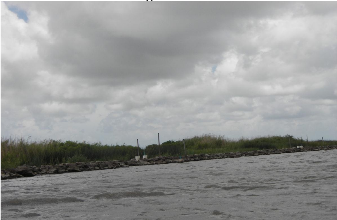
Photo No. 2 , test section
