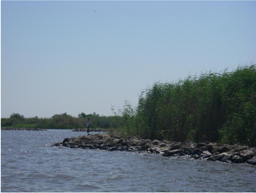
Photo No. 3, Rock Dike on East Shoreline of Grand Lake
