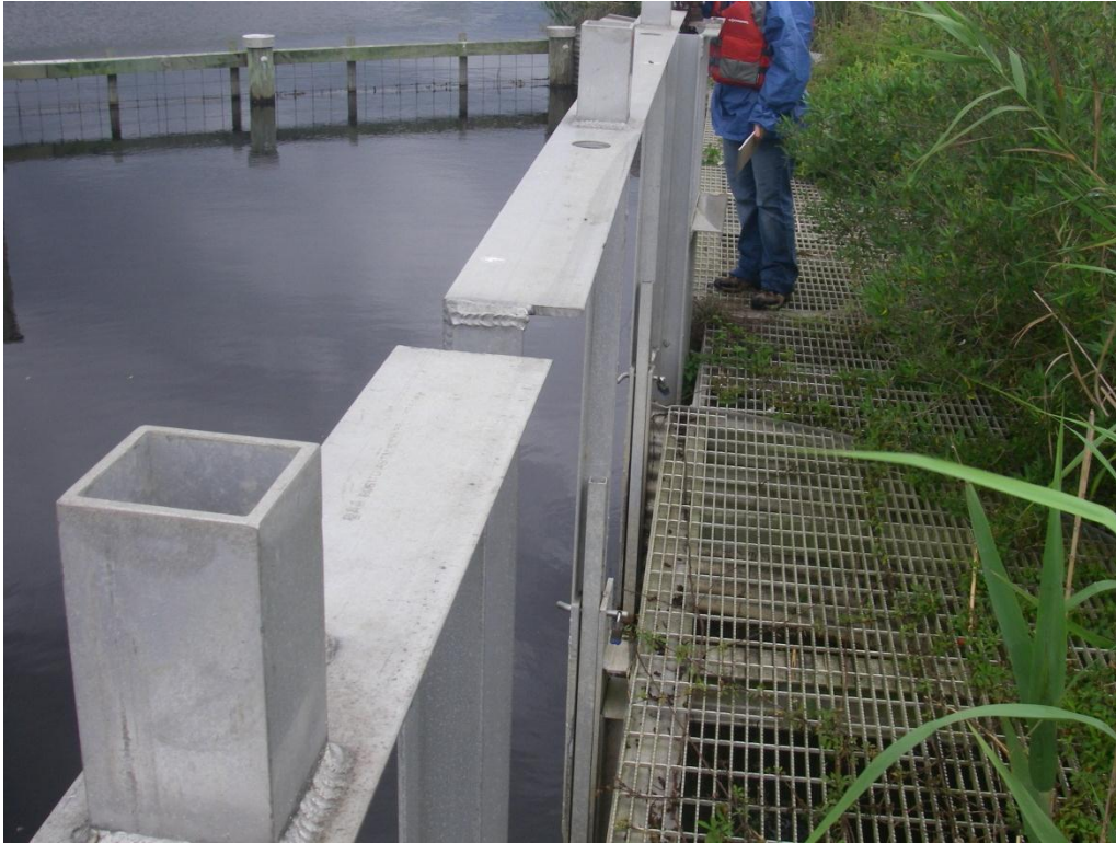
Photo No. 3, Inlet side of structure
