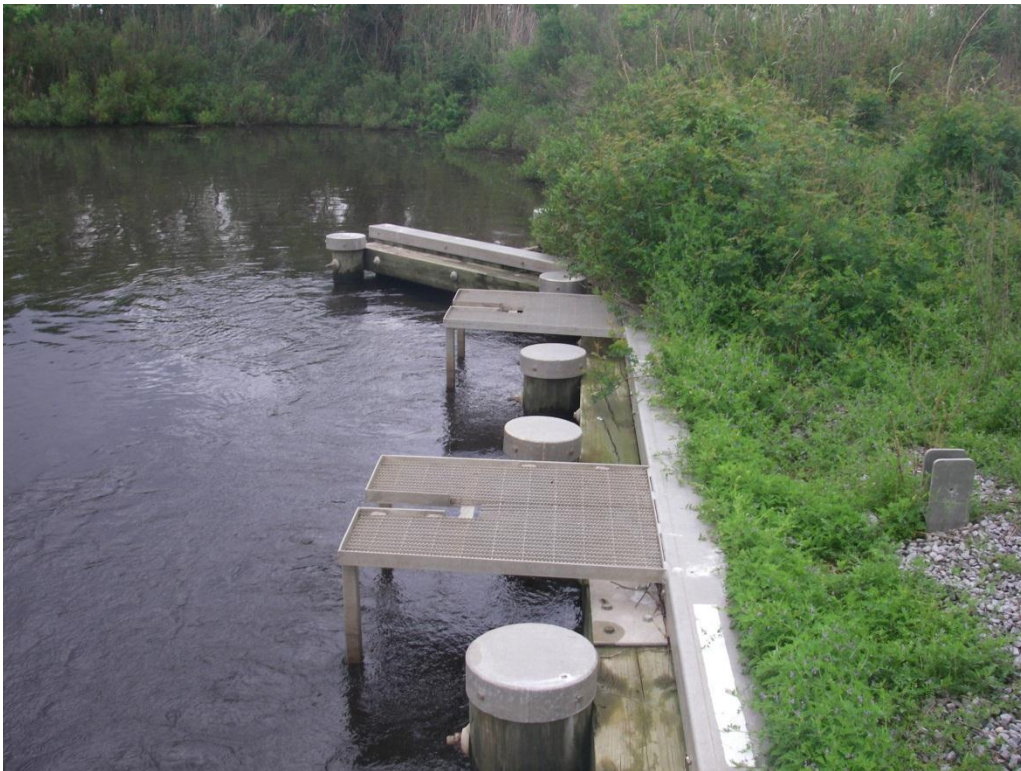
Photo No. 4, Outlet side of structure
