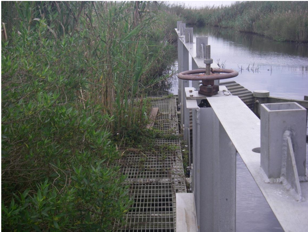
Photo No. 2, Inlet side of structure
