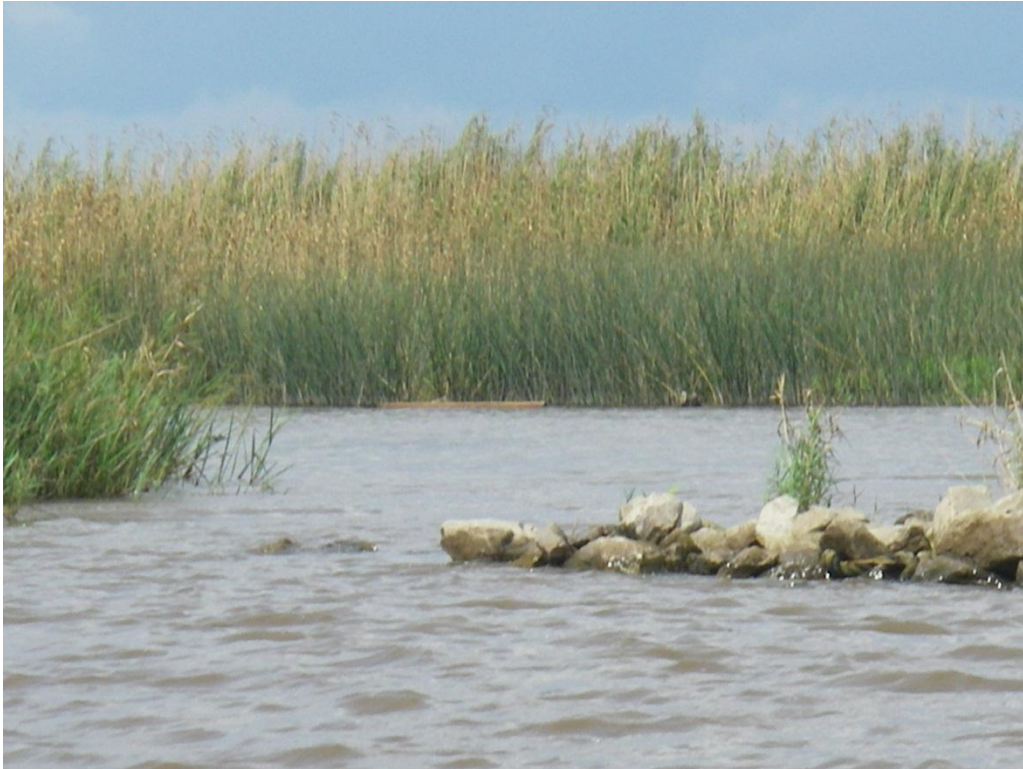
Photo No. 3, Low Area with Displaced Rock
