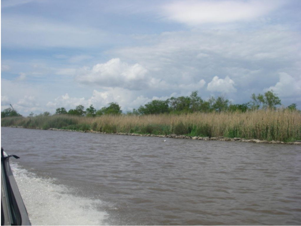
Photo No. 1, (Northern Bank of GIWW) Typical rock dike
