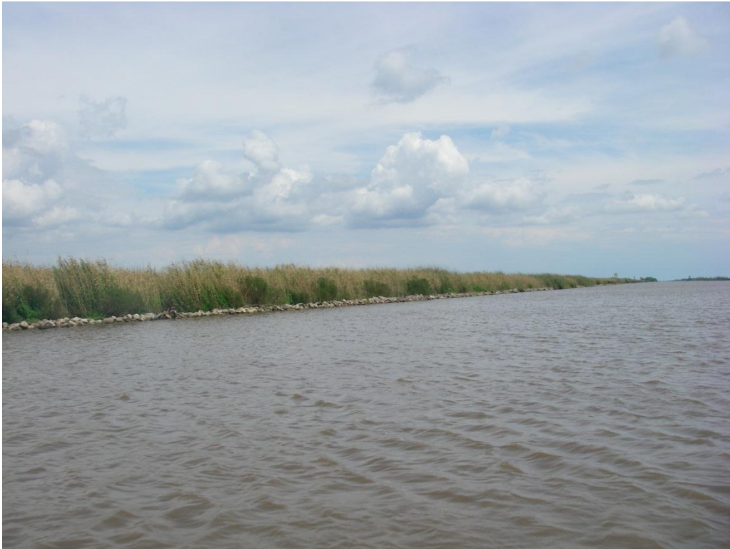
Photo No. 2, (Northern Bank of GIWW) Typical rock dike
