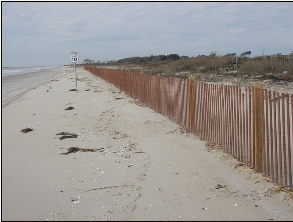
Photo No. 1 , Typical sand fence section
