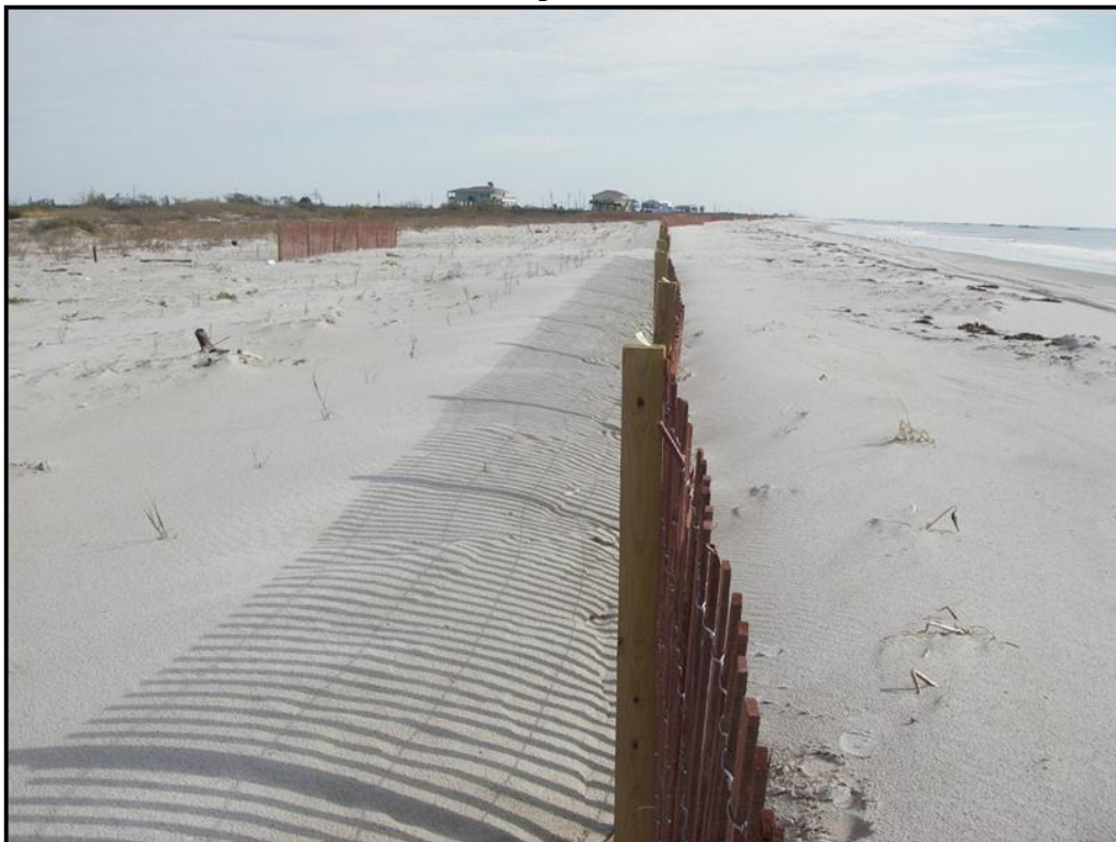
Photo No. 4, Sand collecting on each side of fence beginning to form a dune. Also, plantings can be seen at toe of new dune on northern side of fence.
