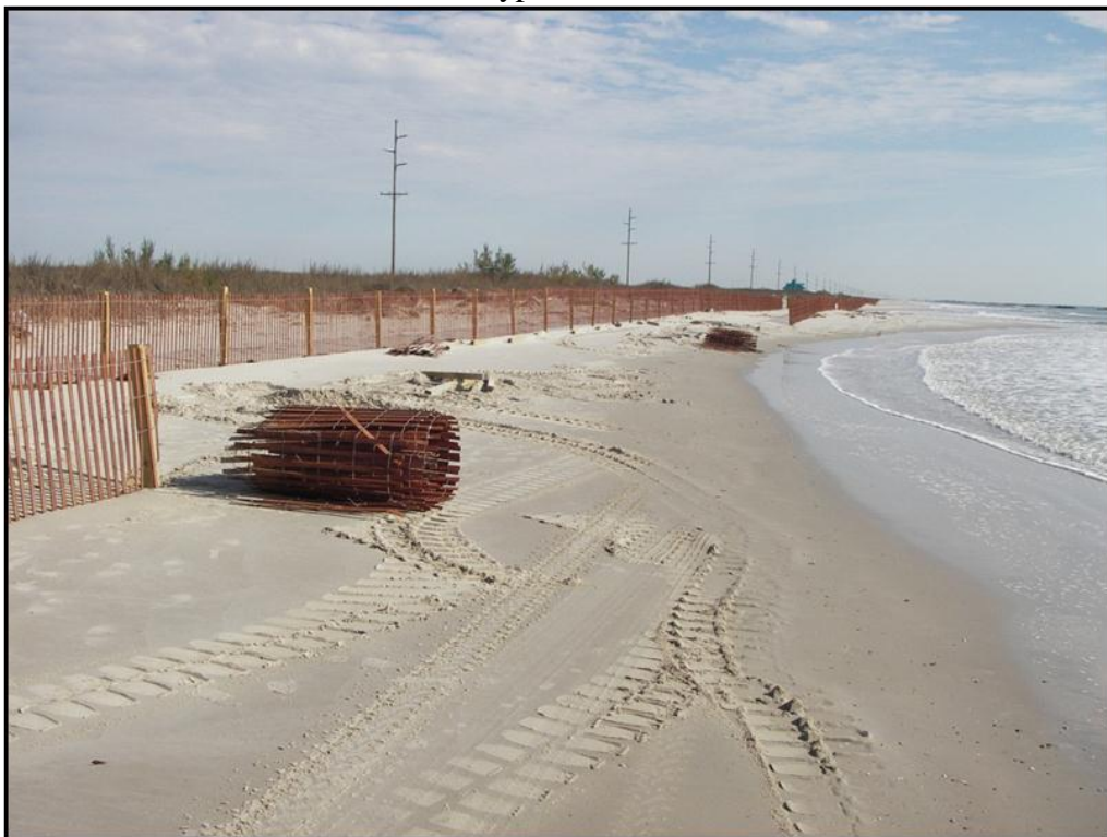
Photo No. 2 , 150 foot section of damaged fence removed
