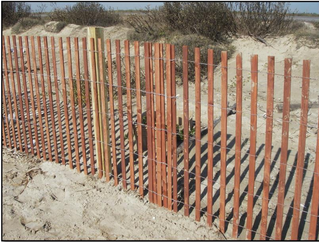
Photo No. 3, Spliced fence section
