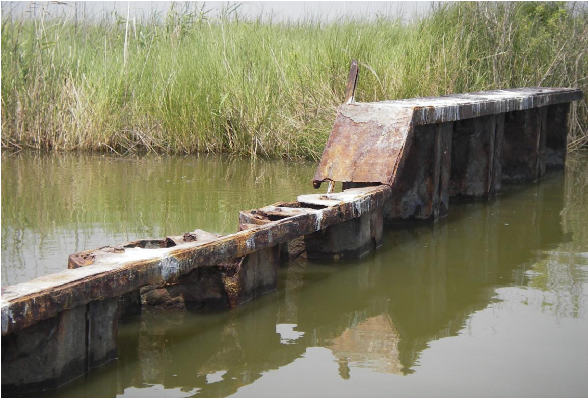
Photo 20, Rusted Sheet Piles on Structure 17
