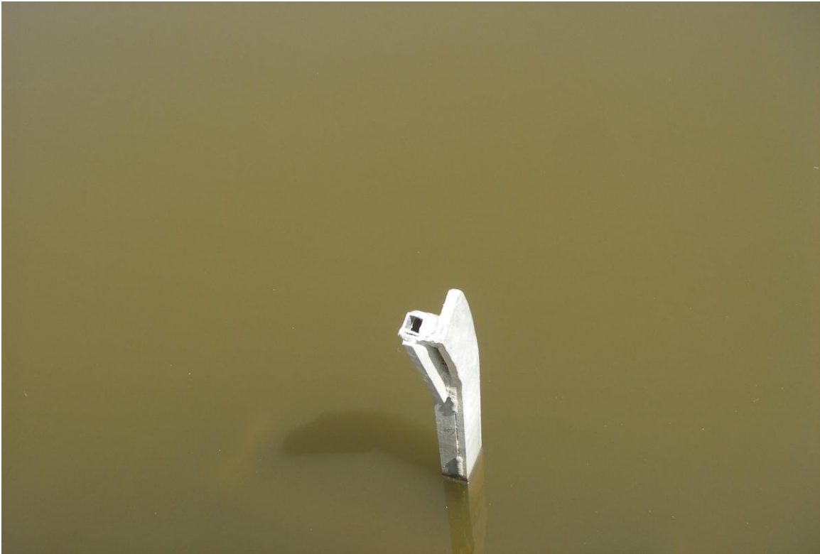
Photo No. 5, Broken Lifting Arm on Structure 9b
