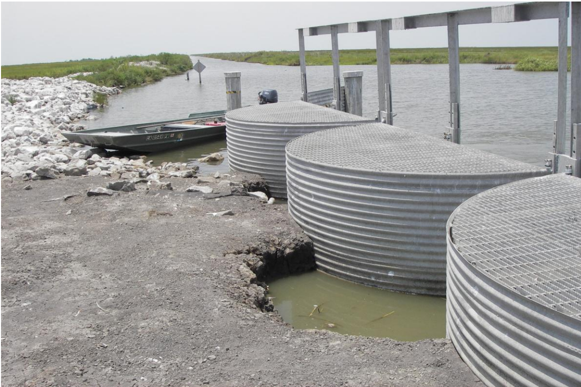
Photo 14, Sinkholes Developing Behind Structure 4 Stoplog Bays
