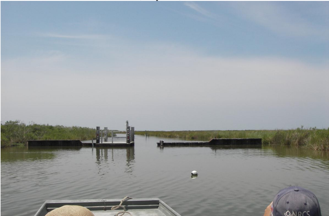
Photo 19, Flanking Around Structure 17
