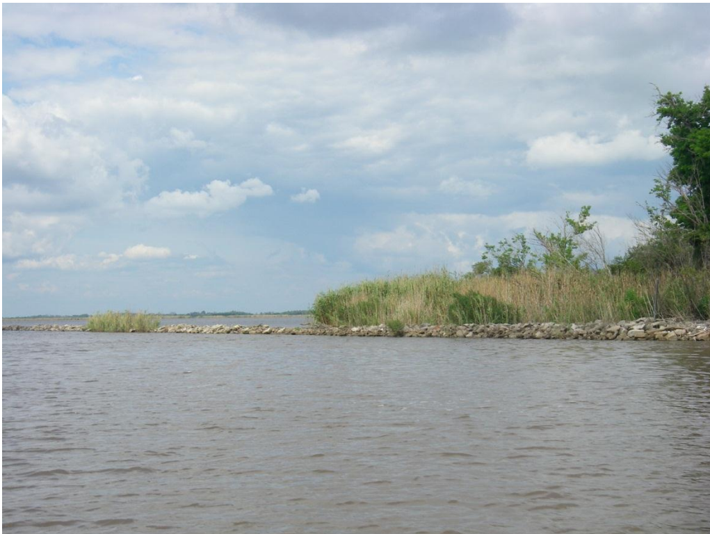
Photo No. 4, Willow Lake Rock Dike (Southeastern End)
