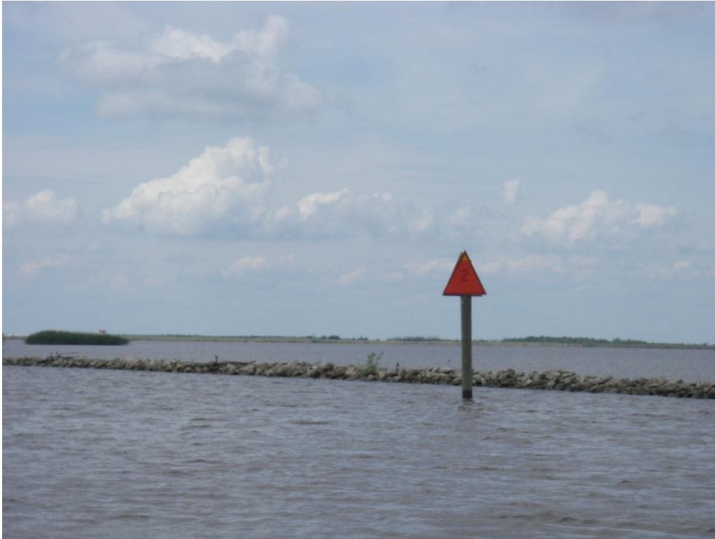
Photo No. 1, (Sweet Lake) Typical rock dike
