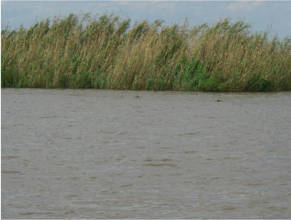
Photo No. 3, Sweet Lake Low Area in Rock Dike
