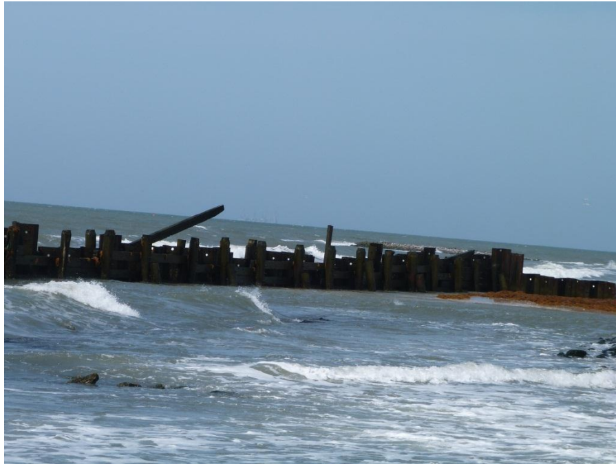
Photo 8: Gulf Shoreline near station 58+00 looking SSW (NOAA #P1000057). Note the timber bulkhead formerly behind the project dune feature now in the gulf shoreline.
