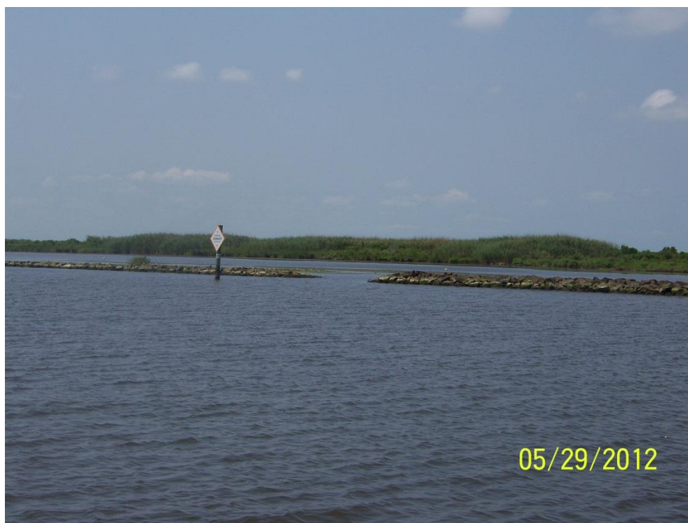
Photo #14: View of fish dip and warning sign between Rock Segments #7 and #8, looking southwest
