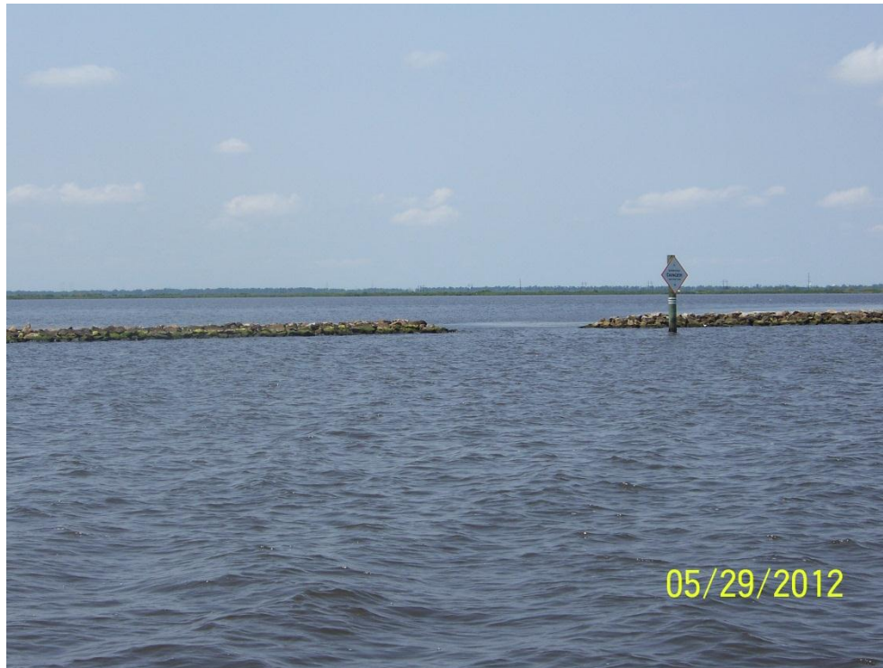
Photo #7: View of fish dip and warning sign between Rock Segment #2 & #3, looking southwest
