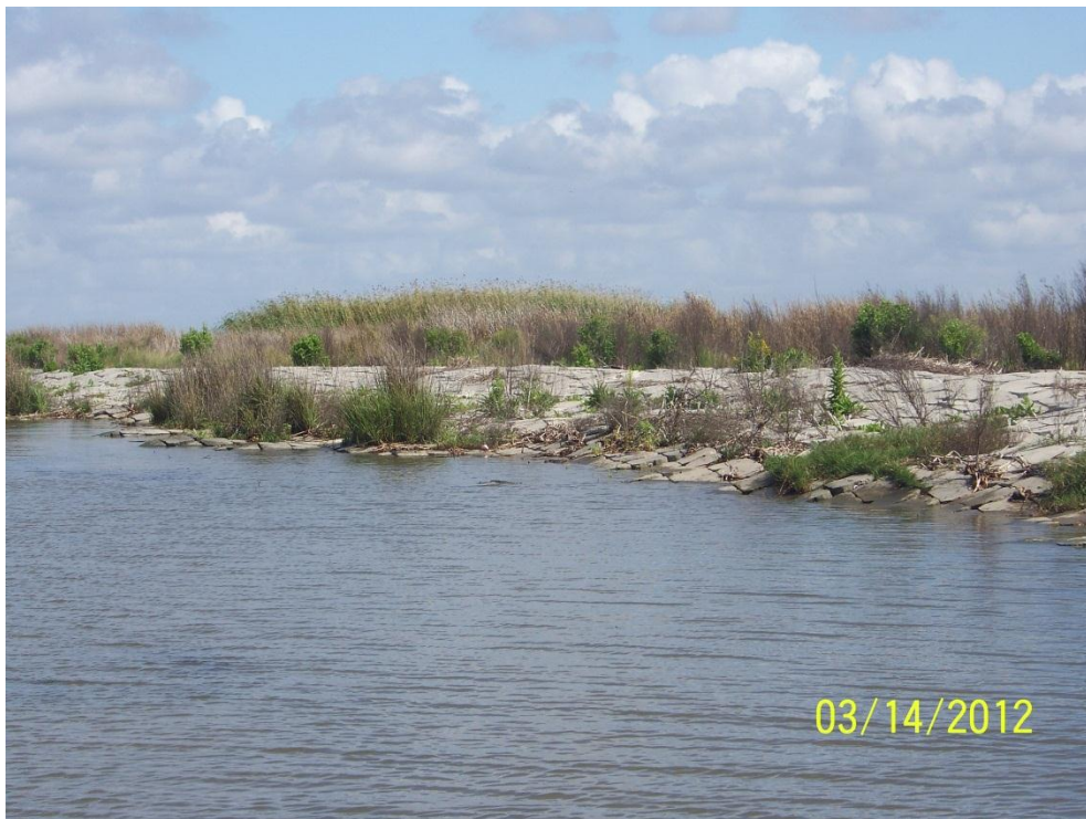
Photo 24: Close up view of articulated concrete mats along Bayou Raccourci, looking east
