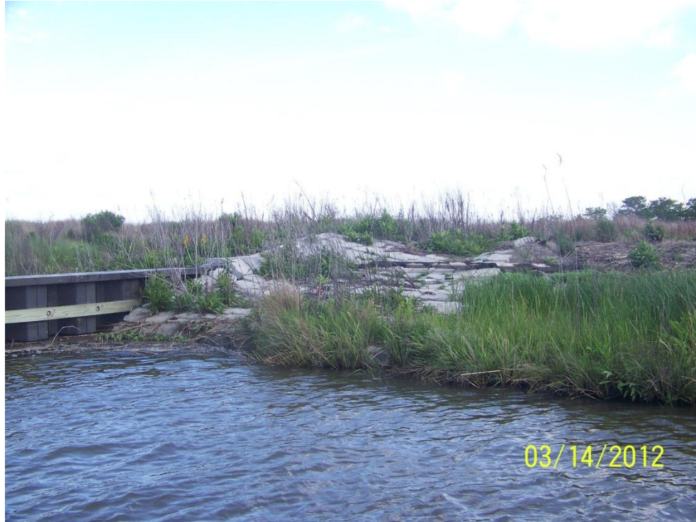
Photo 17: View of articulated concrete mat used to armor the embankment tie-in on Sheetpile Plug 3
