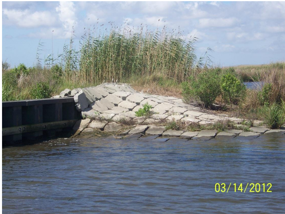
Photo 39: View of the armored earthen embankment tie-in on the western side of Sheetpile Plug 1, looking southwest
