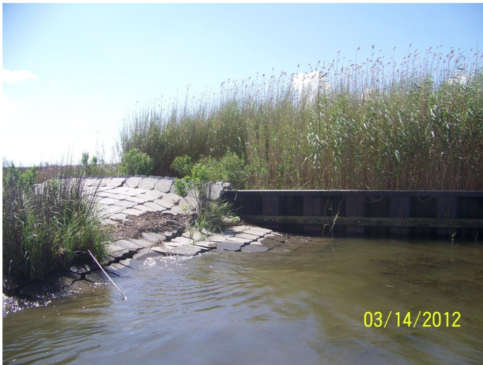
Photo 36: View of the armored earthen embankment tie-in on the eastern side of Sheetpile Plug 1, looking south
