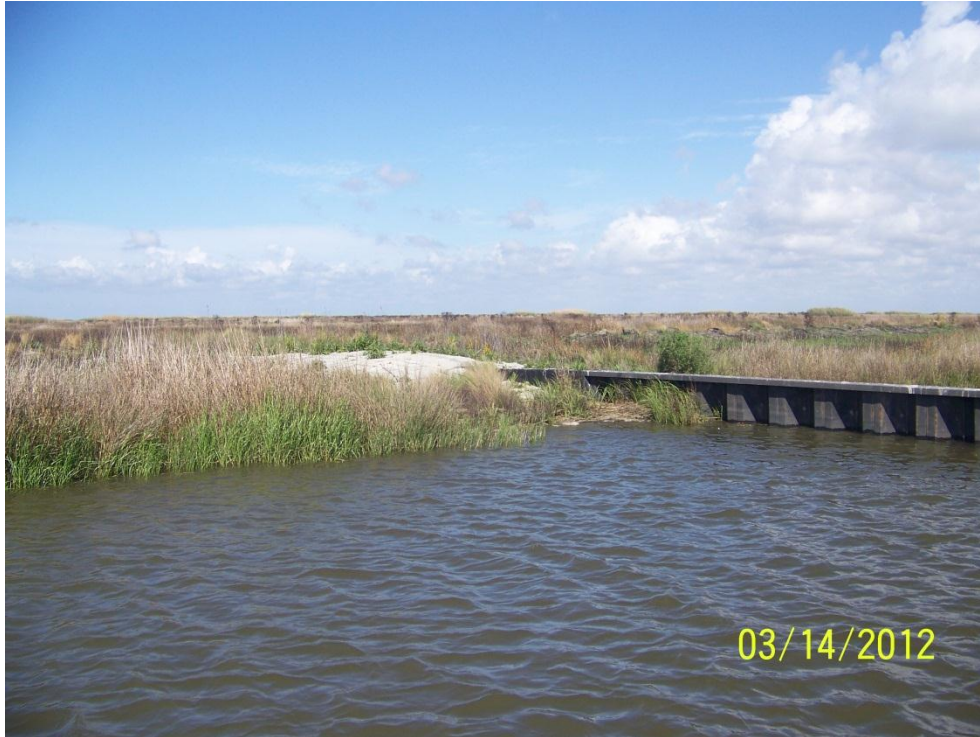
Photo 33: View of the armored earthen embankment tie-in on the west side of Sheetpile Plug 2
