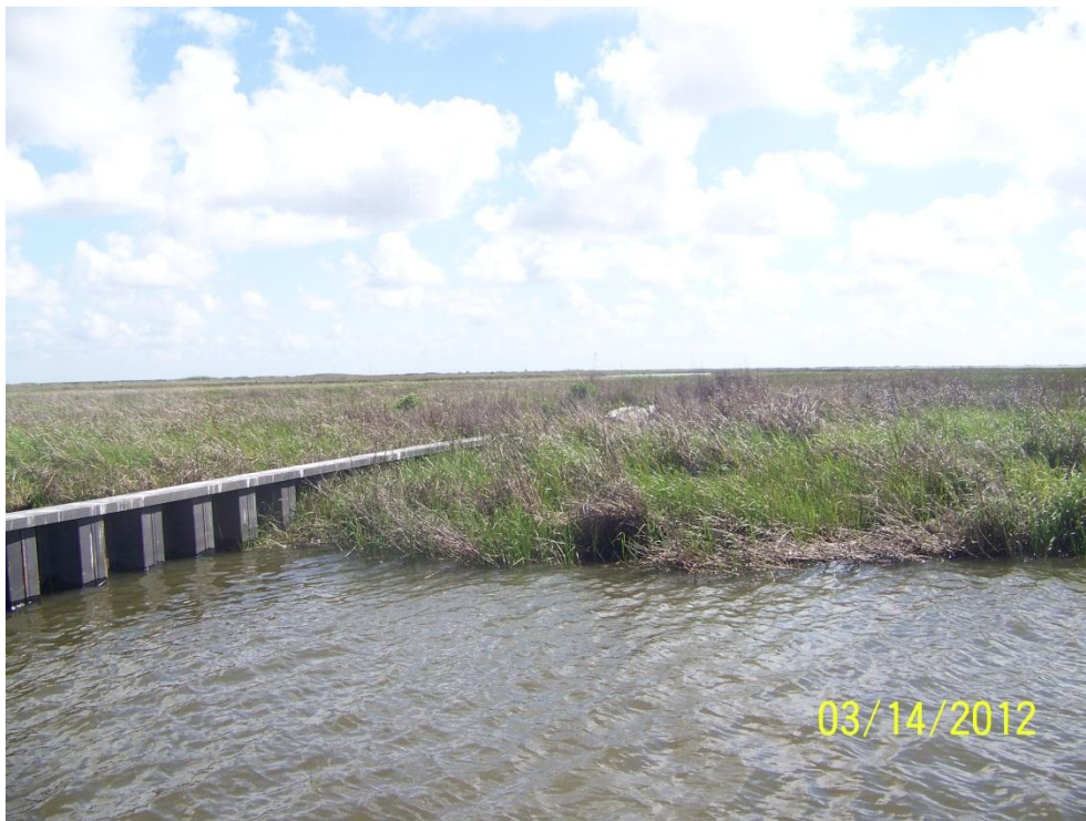
Photo 34: View of the armored earthen embankment tie-in on the east side of Sheetpile Plug 2
