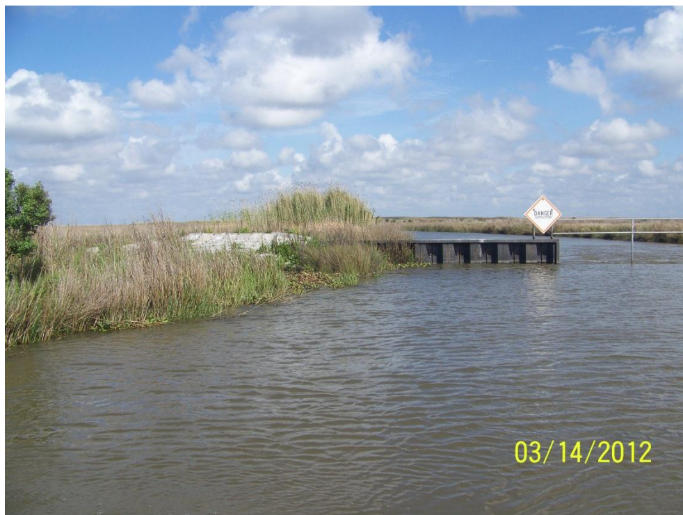
Photo 28: View of the Sheetpile Weir embankment tie-in on the west side, looking north
