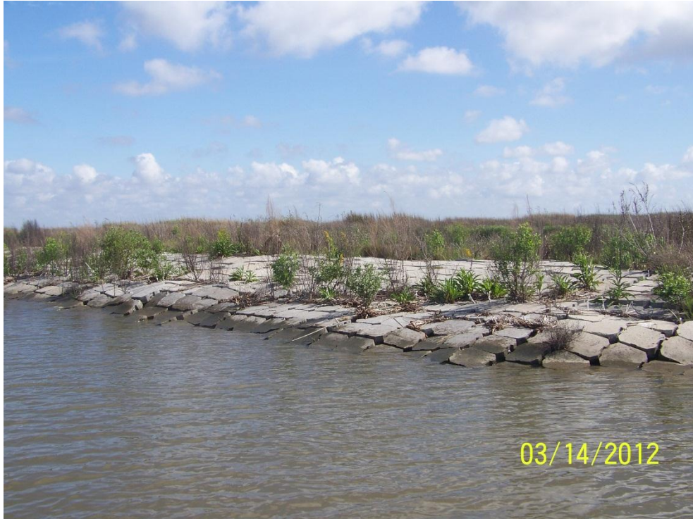
Photo 23: Close up view of articulated concrete mats along Bayou Raccourci, looking east
