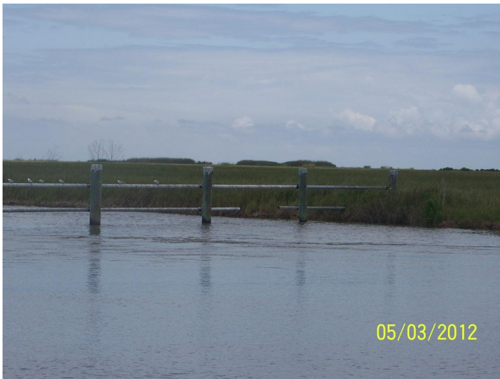
Photo #24: View of missing section on interior barricade system of Site No. 4, looking west.
