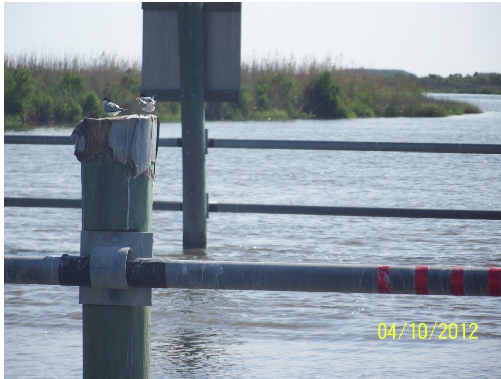
Photo #7: Visible corrosion of galvanized end caps on the timber barricade supports in Site No. 9
