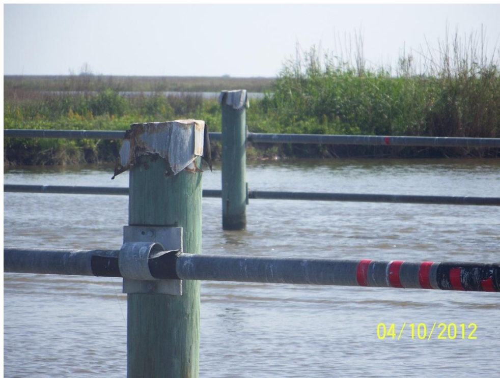
Photo #6: Visible corrosion of galvanized end caps on the timber barricade supports in Site No. 9
