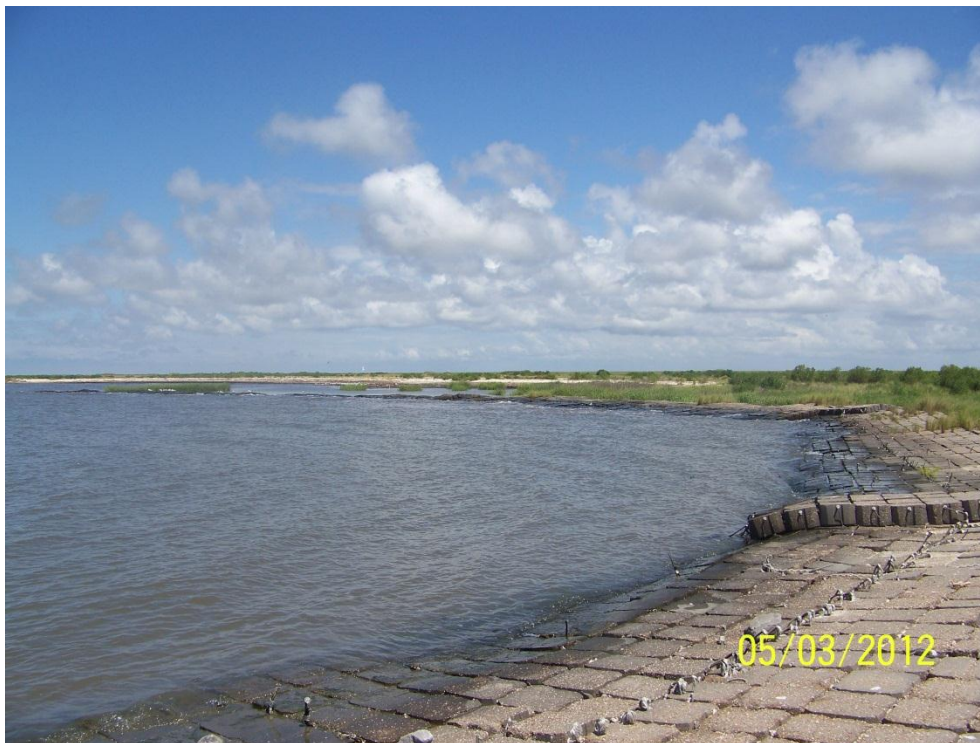
Photo No. 34: View of the articulated concrete mats on the western end of the Transco Canal rock dike, looking east
