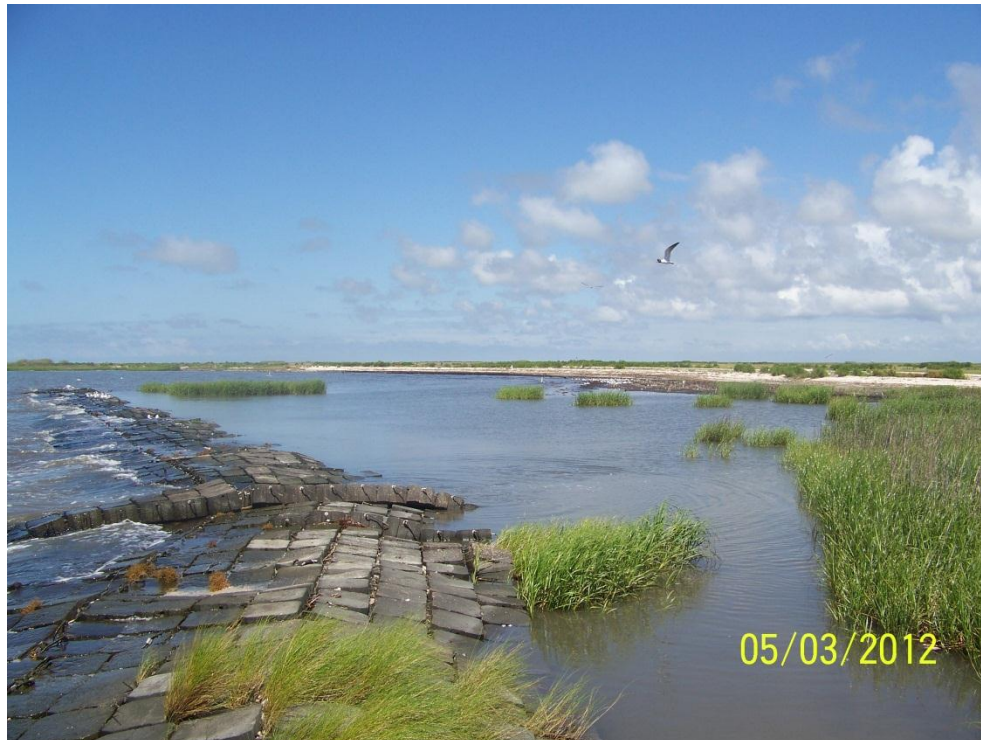
Photo No. 35: View of erosional shadowing behind the end of the articulated concrete mats on the western end of the Transco Canal rock dike, looking east
