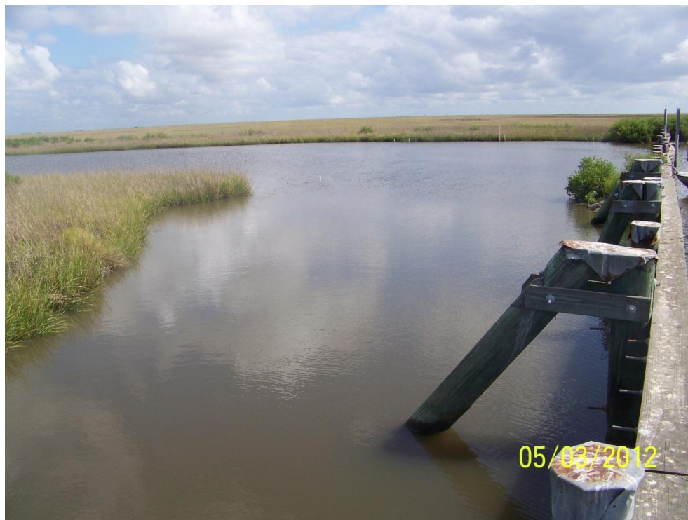
Photo No. 12: View of the breach around the southern end of Plug No. 8 from the western side of the structure, looking north
