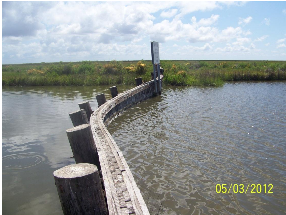
Photo No. 25: View of the timber bulkhead deflection on Plug No. 6 from on top of the structure, looking east
