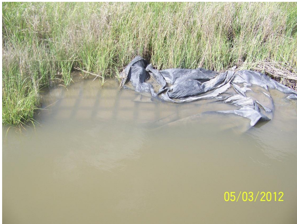
Photo No. 9: View of the Submar scour mats placed on the southern end of Plug No. 8 from on top of the structure, looking south
