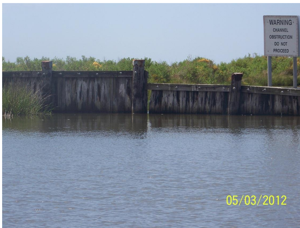
Photo No. 24: View of a separation in the timber bulkhead of Plug No. 6 from Transco Canal, looking south
