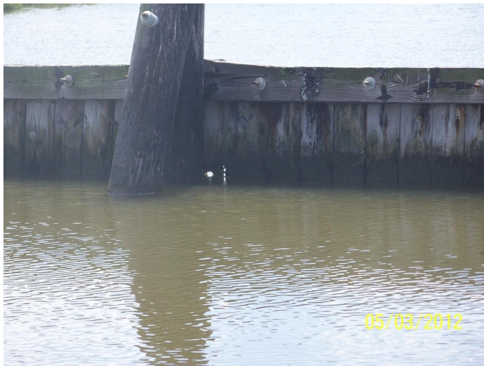
Photo No. 20: View of deteriorated timber boards along the waterline on Plug No. 7, looking east
