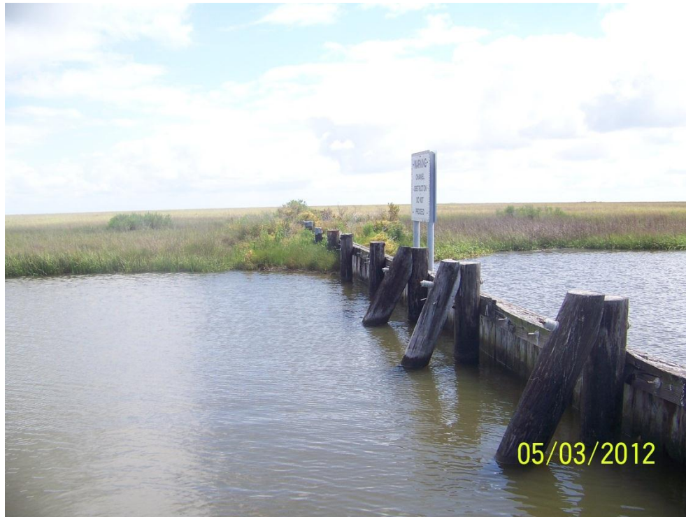
Photo No. 21: View of batter piles on the western side of Plug No. 7, looking north
