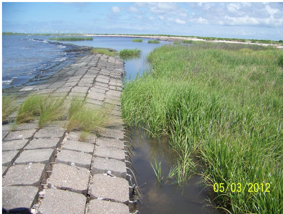
Photo No. 36: View of water wrapping around the articulated concrete mats, looking east. The water has no progressed far enough to reach Transco Canal.
