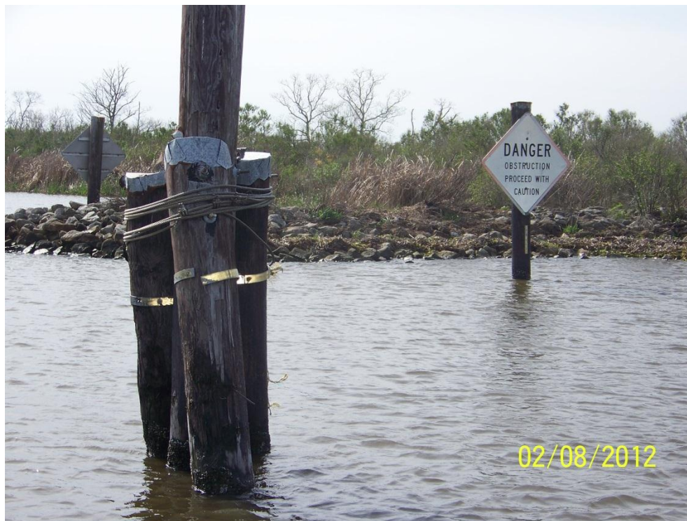
Photo #12: Close up view of damaged timber dolphin at Structure 1 to be replaced in the 2012 Maintenance Project
