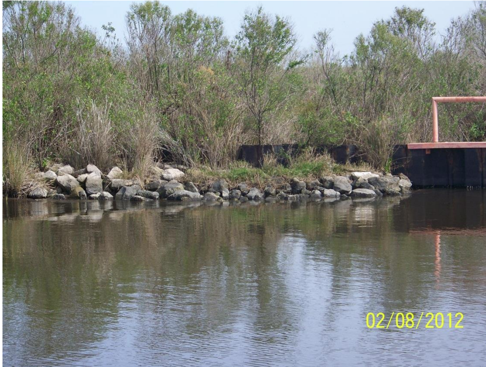
Photo #27: View of embankment tie-in on the northwest end of Structure 35
