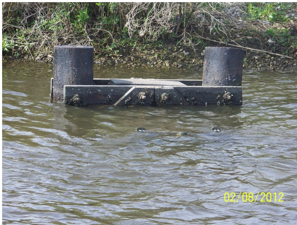
Photo #18: Close up view of Structure 91 culvert protruding above the waterline
