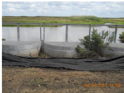
Photo 24 – Geotextile fabric
