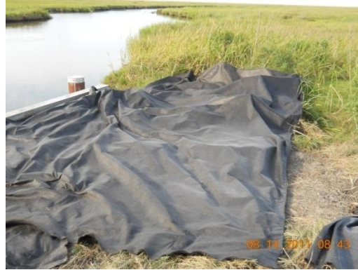
Photo 14 – Geotextile fabric
