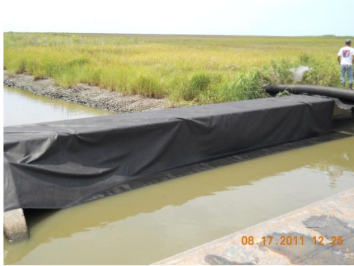
Photo 43 – Geotextile fabric
