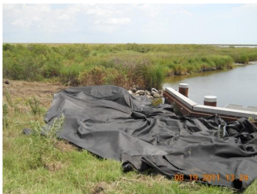
Photo 33 – Geotextile fabric
