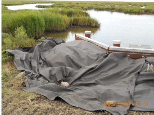
Photo 25 – Geotextile fabric
