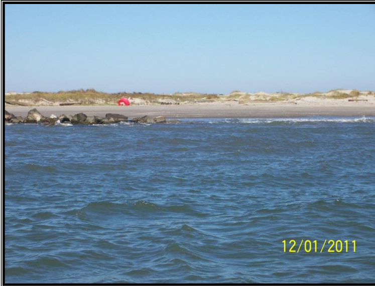
Photo 21 Site #6 near station 97+00 looking north at east end of Canal 19 rocks. Note typical erosion pocket at end of rocks, but very little erosion noted at east end of project. Large dunes remain with evidence of newly deposited sand.
