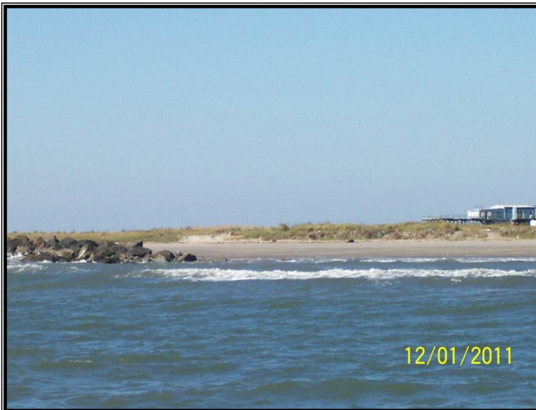
Photo 20. Site #5 near station 107+00 looking northwest at east end of Canal 19 rocks. Note typical erosional shadow behind end of rocks, but overall little erosion on the west end of the project.
