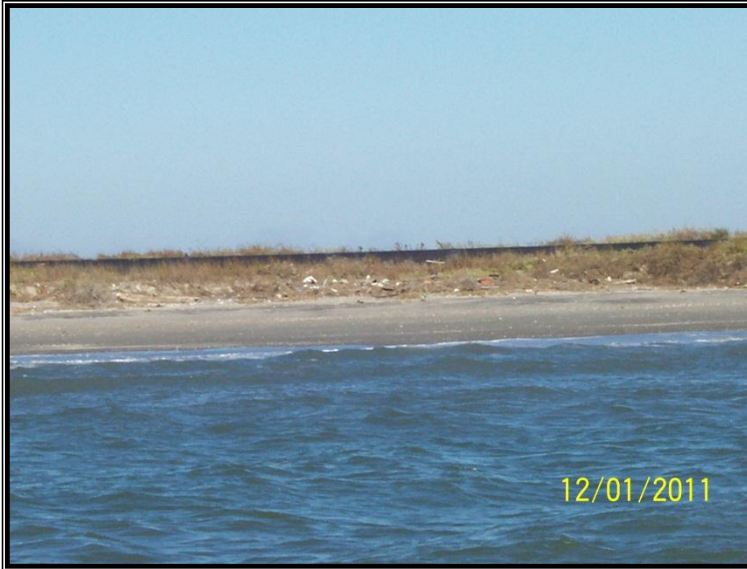
Photo 13. Site #4 near station 122+00 looking north. Note wider beach with less scarping of the dune. Dune feature is wider with good vegetative cover.
