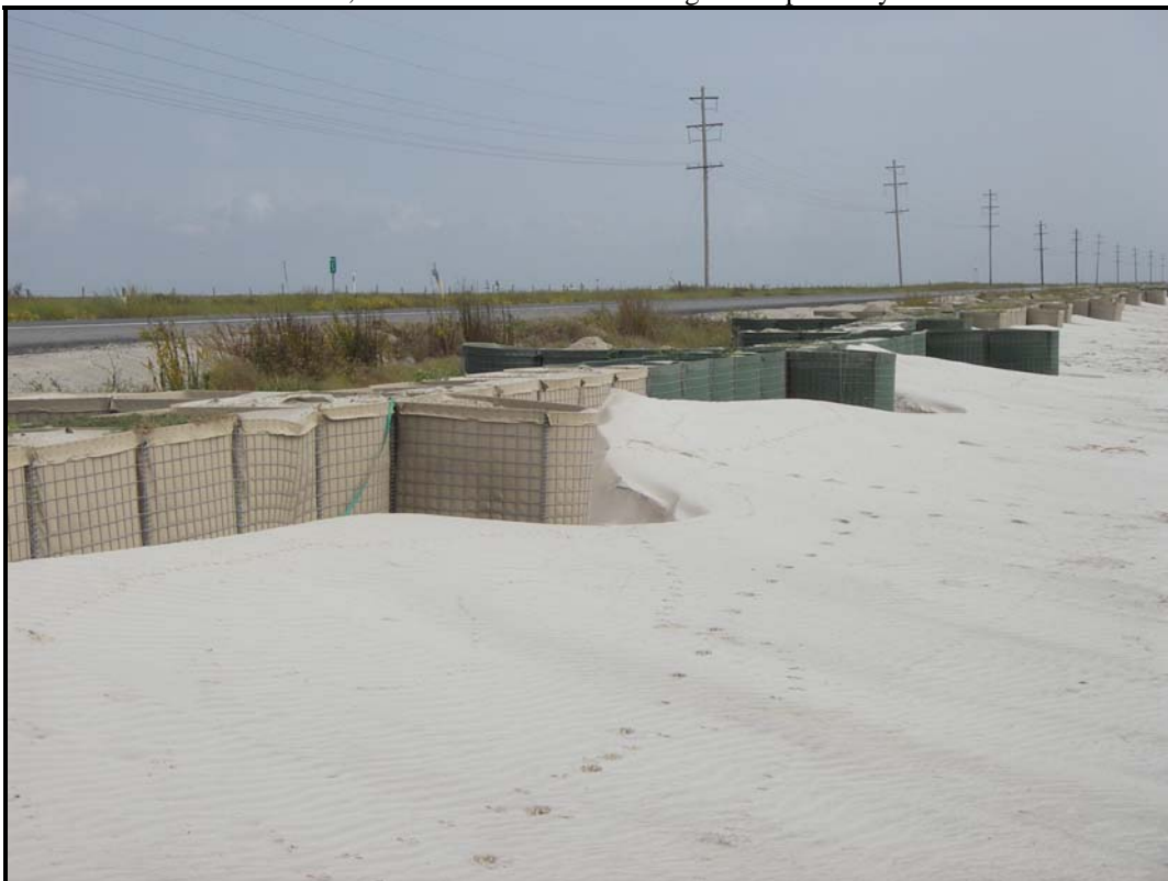
Photo No. 4, View of HESCO Baskets trapping sand, looking eastward
