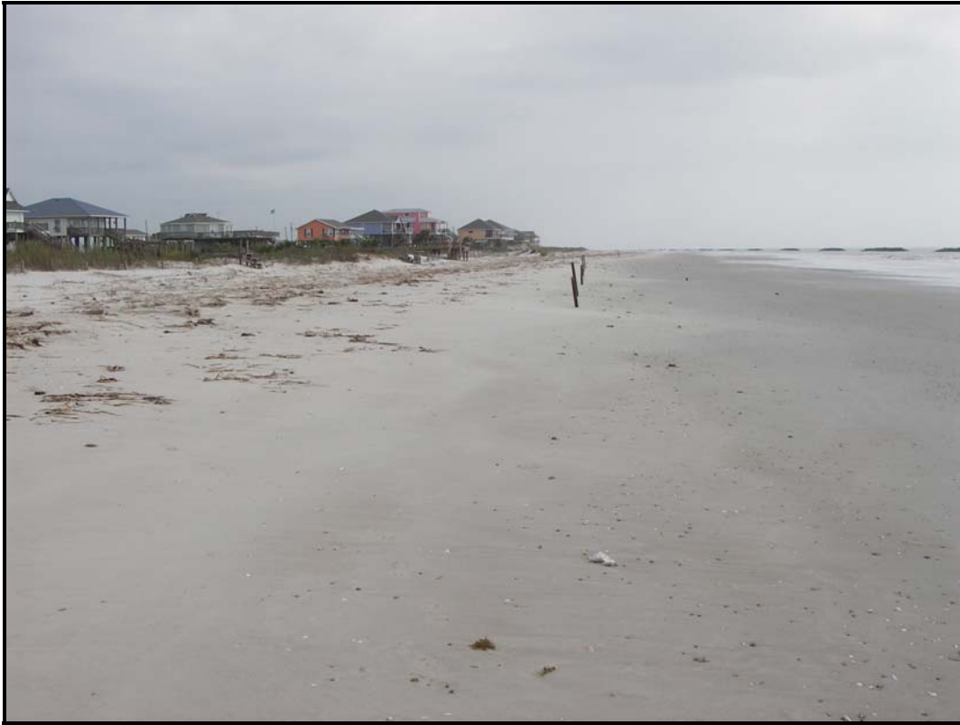
Photo No. 1, Typical view of destroyed sand fence and erosion to beach
