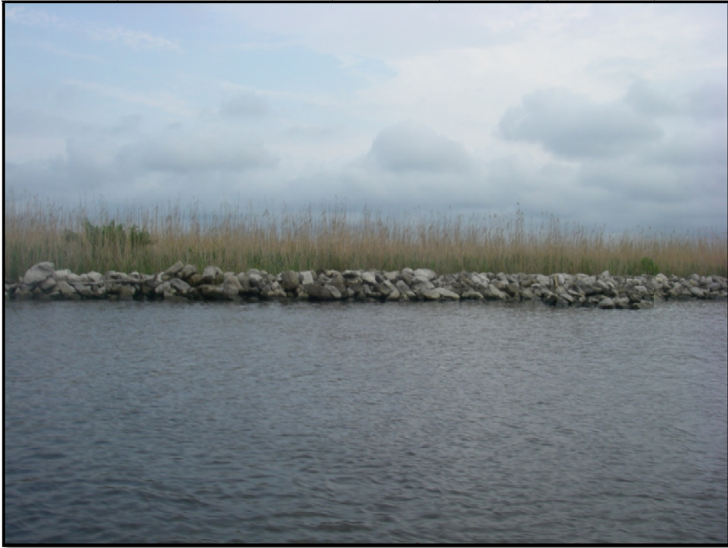
Photo No. 1, Typical rock dike
