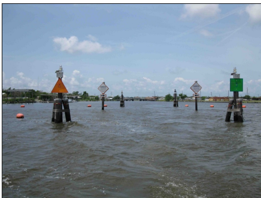
Photo 2. Naomi Outfall Management (BA-03c). Goose Bayou Canal weir, looking west. The weir has settled below the waterline.
