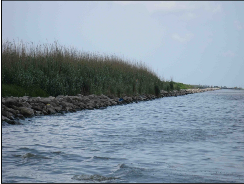
Photo 5. Evidence of accretion behind the rock wall for the BA-26 project.
