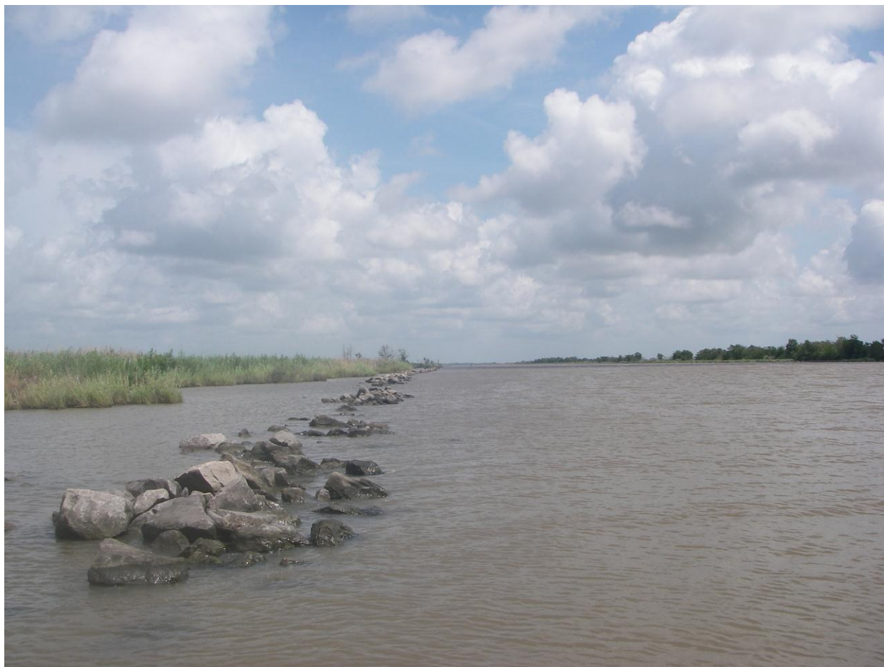
Figure 7. Another view looking north at settled rock along Freshwater Bayou Canal in the ME-13 project area on 30 July 2009.
