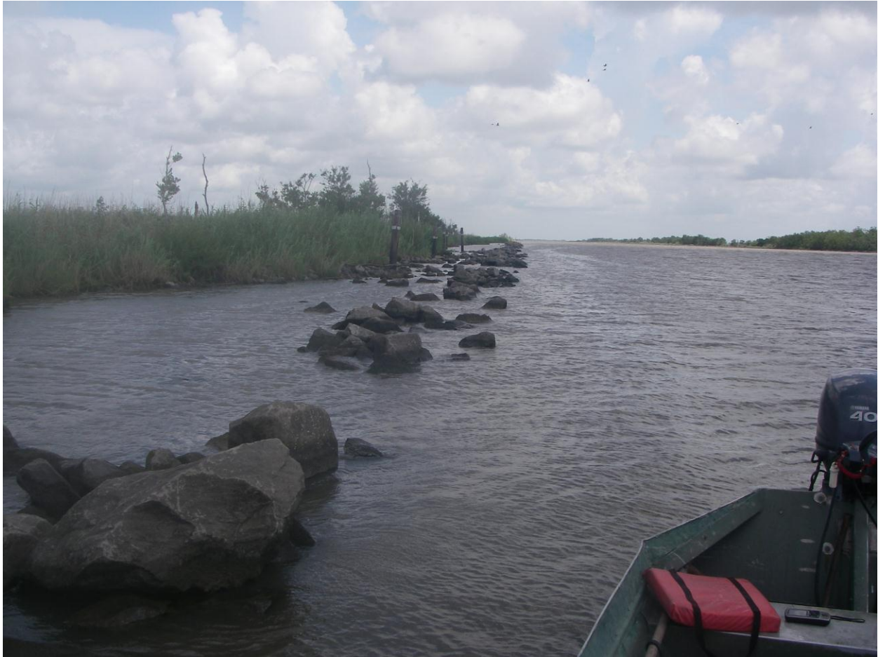
Figure 6. Looking north at settled rock along Freshwater Bayou Canal in the ME-13 project area on 30 July 2009.
