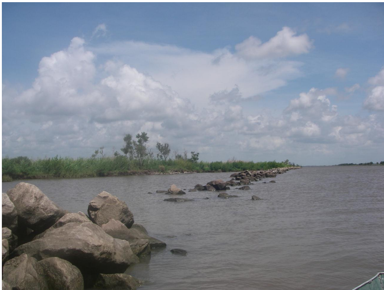
Figure 8. A breach in the settled rock along Freshwater Bayou Canal in the ME-13 project area on 30 July 2009.
