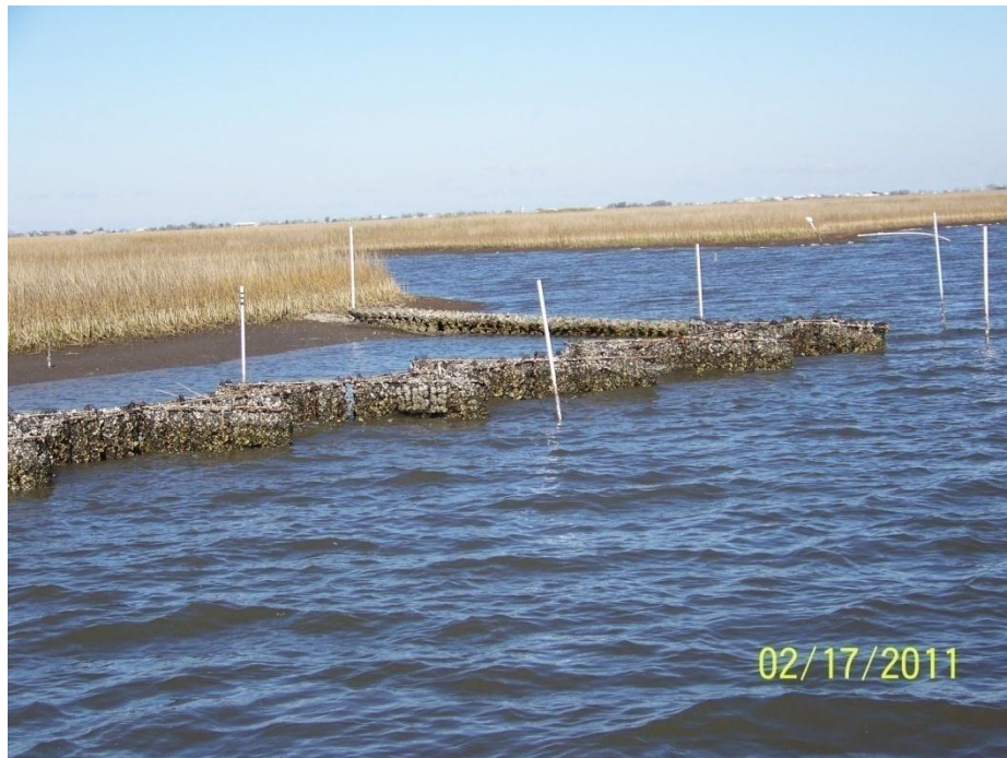
Reach B: ReefBlks and A-Jacks Tie-in to shoreline
