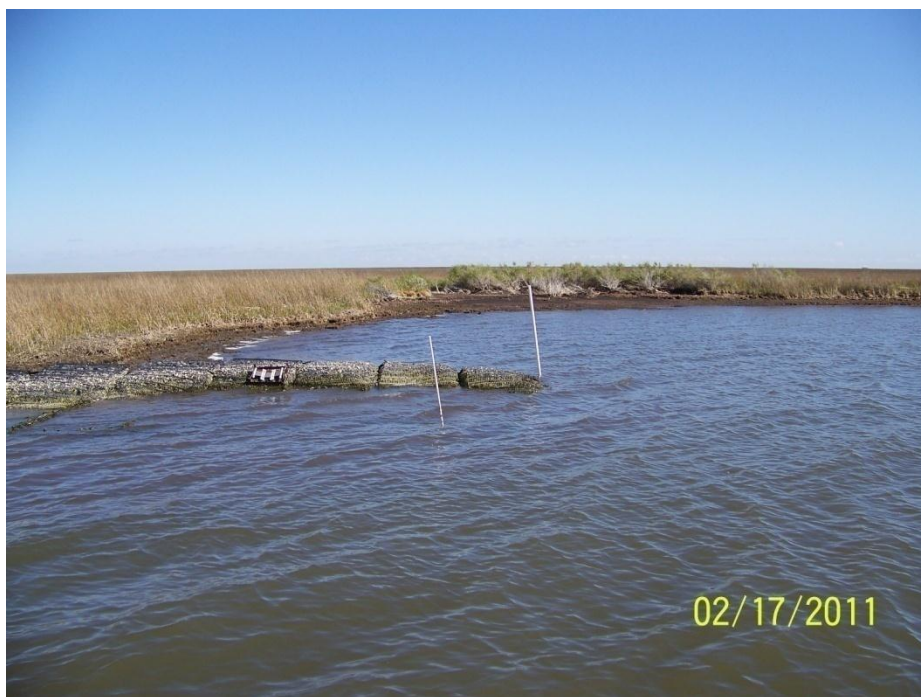
Reach E: Oil damage behind Gabion Mats on South end of section
