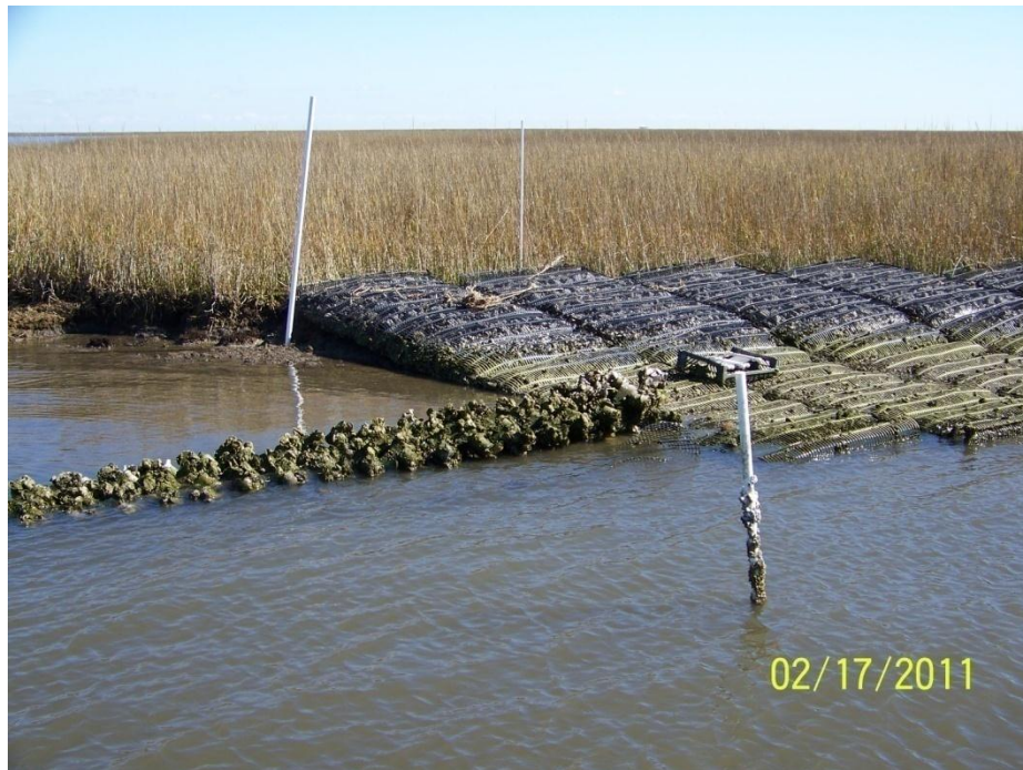
Reach E: A-Jacks tie-in to Gabion Mats
