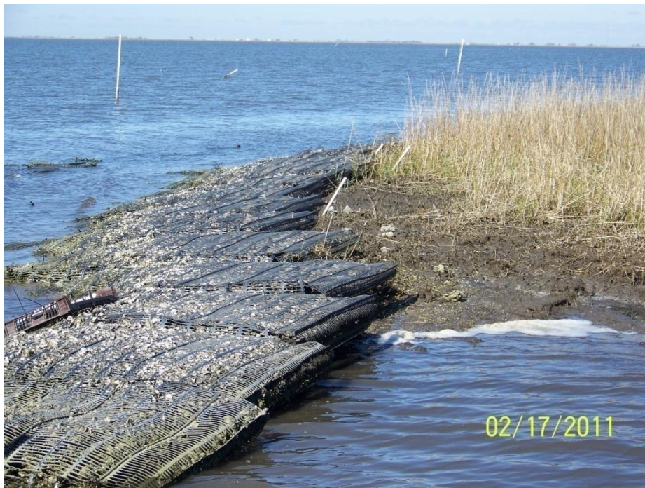
Reach E: Due to oil damage, Gabion mats no longer follow shoreline
