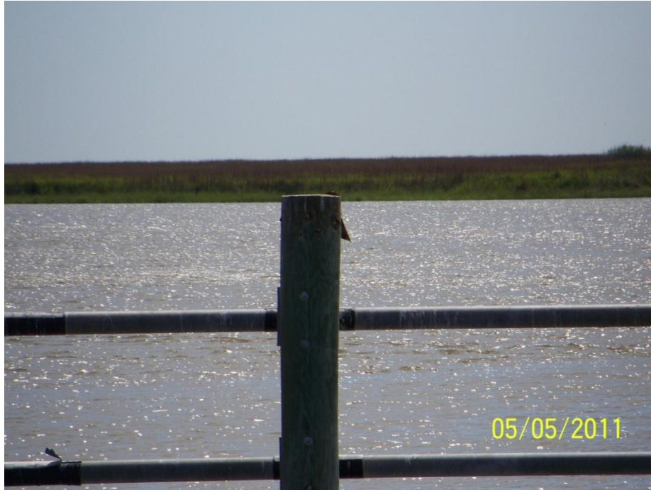
Photo #11: Close up view of missing piling cap on support timber of Site No.9, looking east
