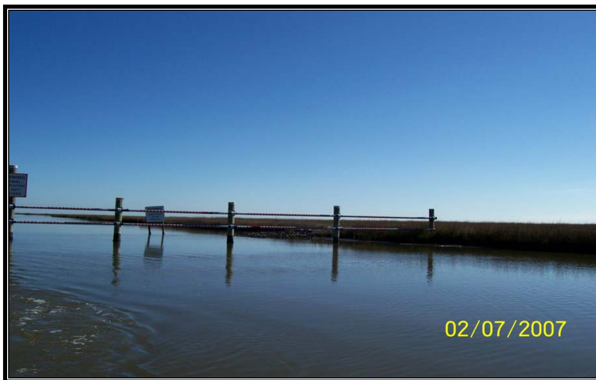
Photo 2 - (Structure No. 1) - Rock weir and timber barricade structure looking east.
