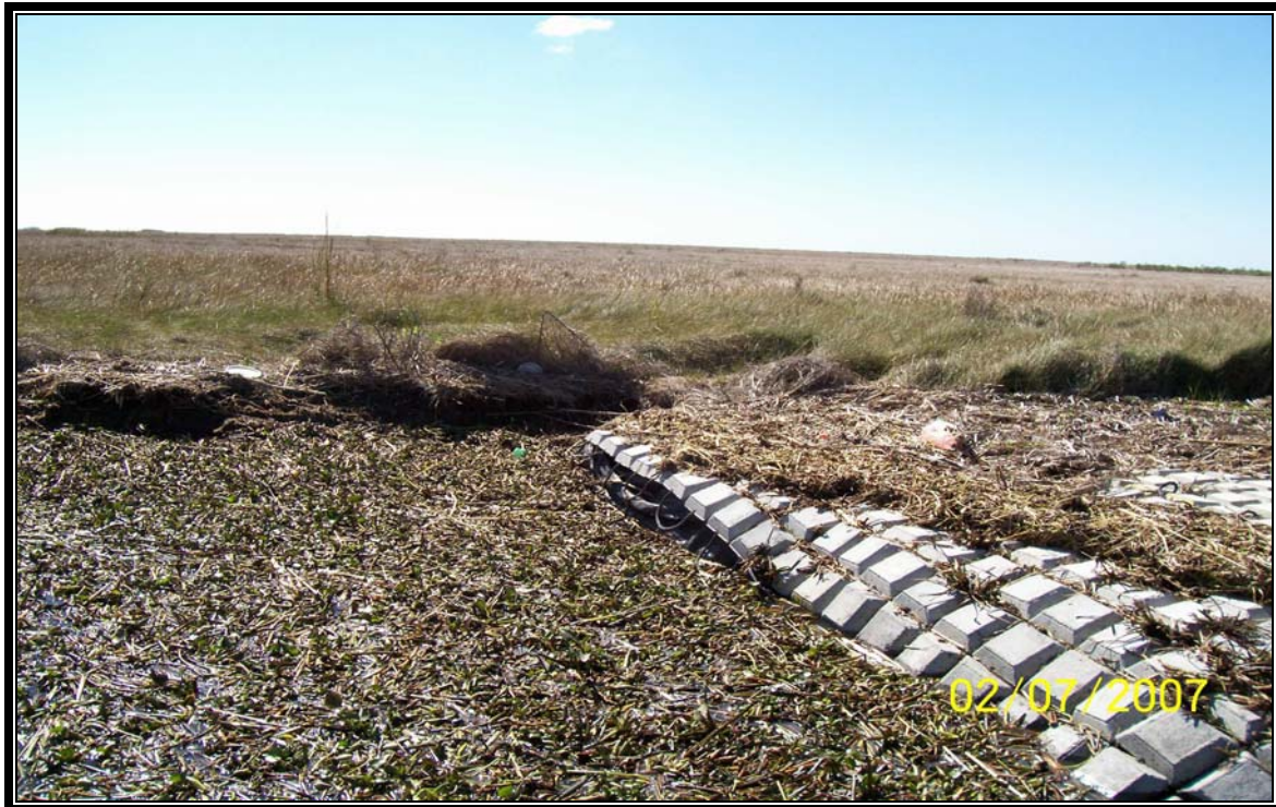
Photo 5 – (Structure No. 3) – Articulated concrete mats tie-in to marsh on south side.
