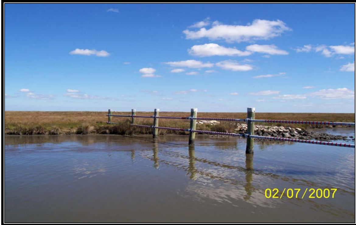
Photo 15 – (Structure No. 6) – Rock weir and timber barricade system looking northeast.
