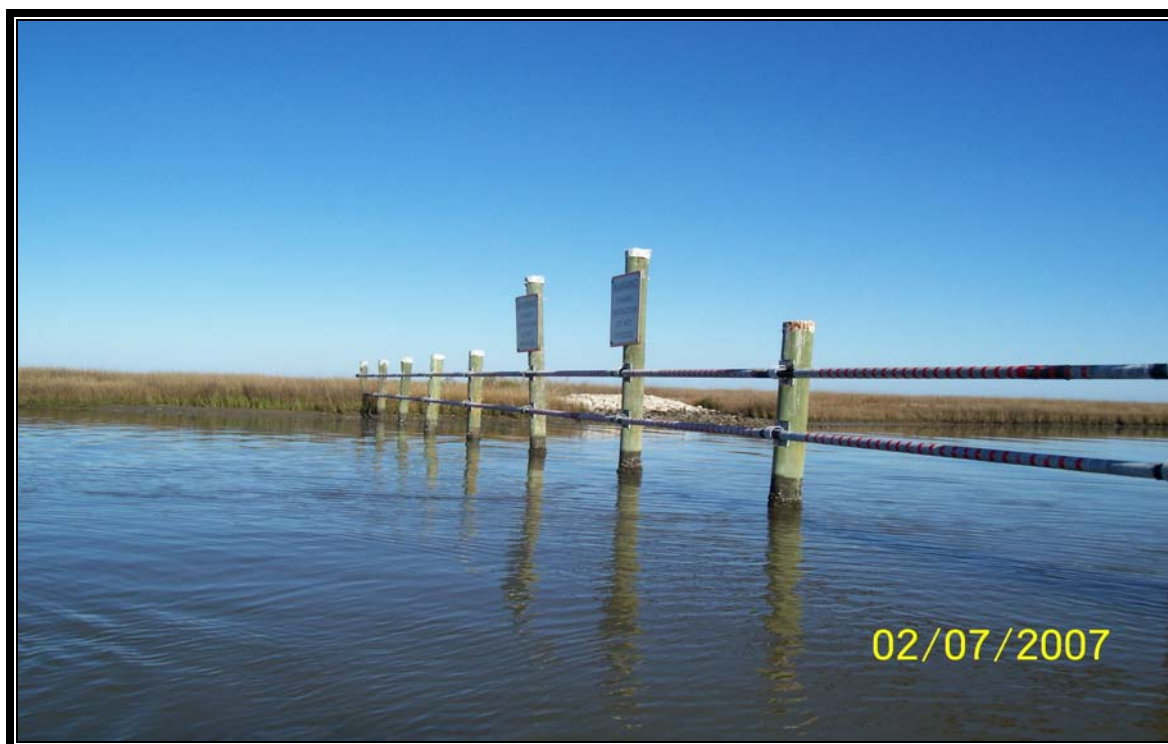
Photo 1 - (Structure No. 1) - Rock weir and timber barricade structure looking north.
