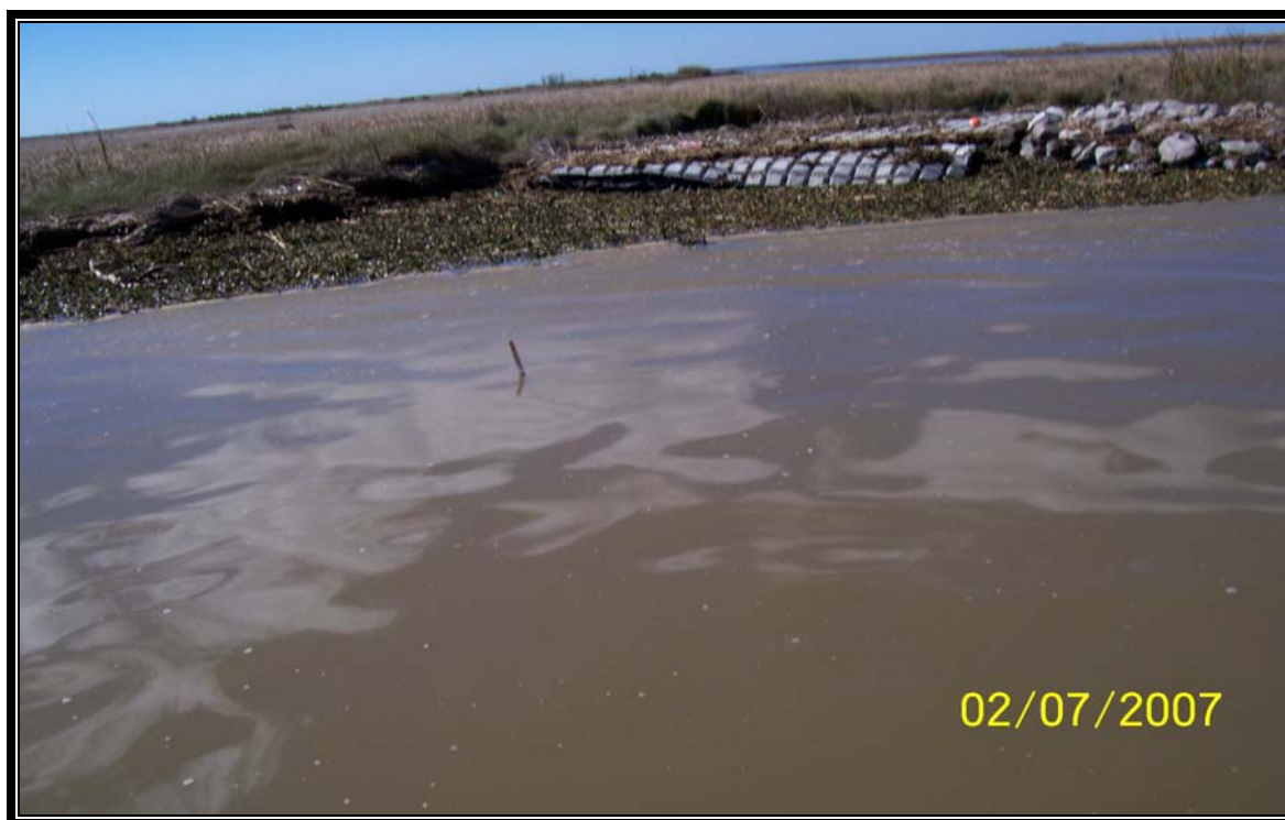
Photo 4 – (Structure No. 3) – Articulated concrete mats tie-in to marsh on south side.
