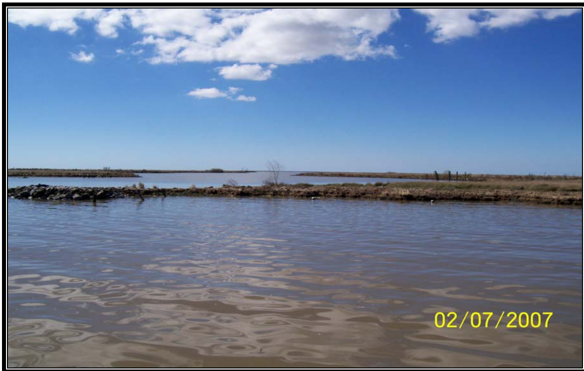
Photo 8 – (Structure No. 3) – Rock weir tie-in to marsh on the north side of the structure.
