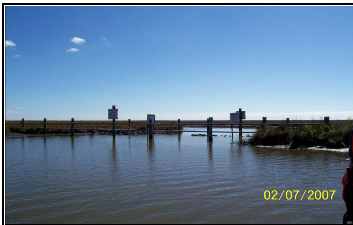
Photo 13 – (Structure No. 5) – Rock weir and timber barricade system looking southeast.
