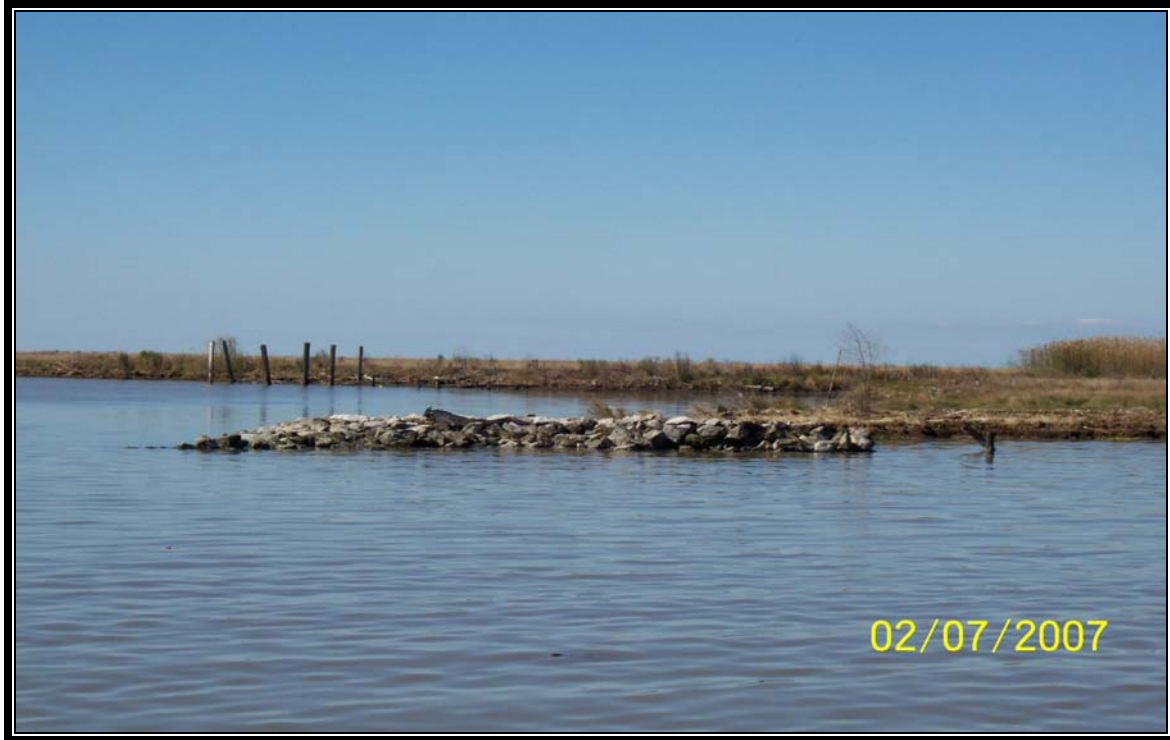
Photo 7 – (Structure No. 3) – Rock weir tie-in to marsh on the north side of structure.
