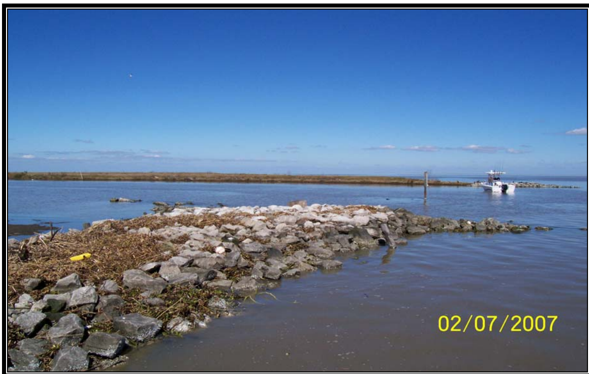
Photo 6 – (Structure No. 3) – Rock weir on the south side of the structure.
