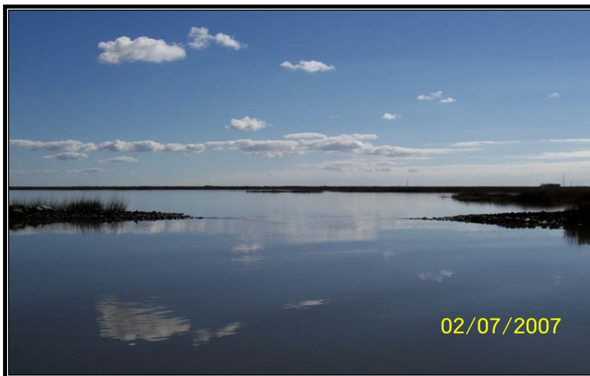
Photo 23 – (Breach 3) – Breach in rock lined bank along oilfield canal.
