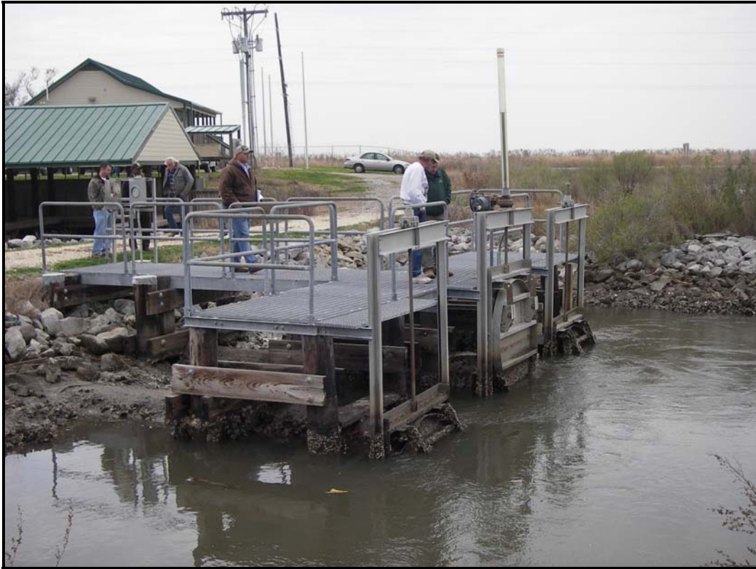
Photo No. 3, Headquarters Structure
