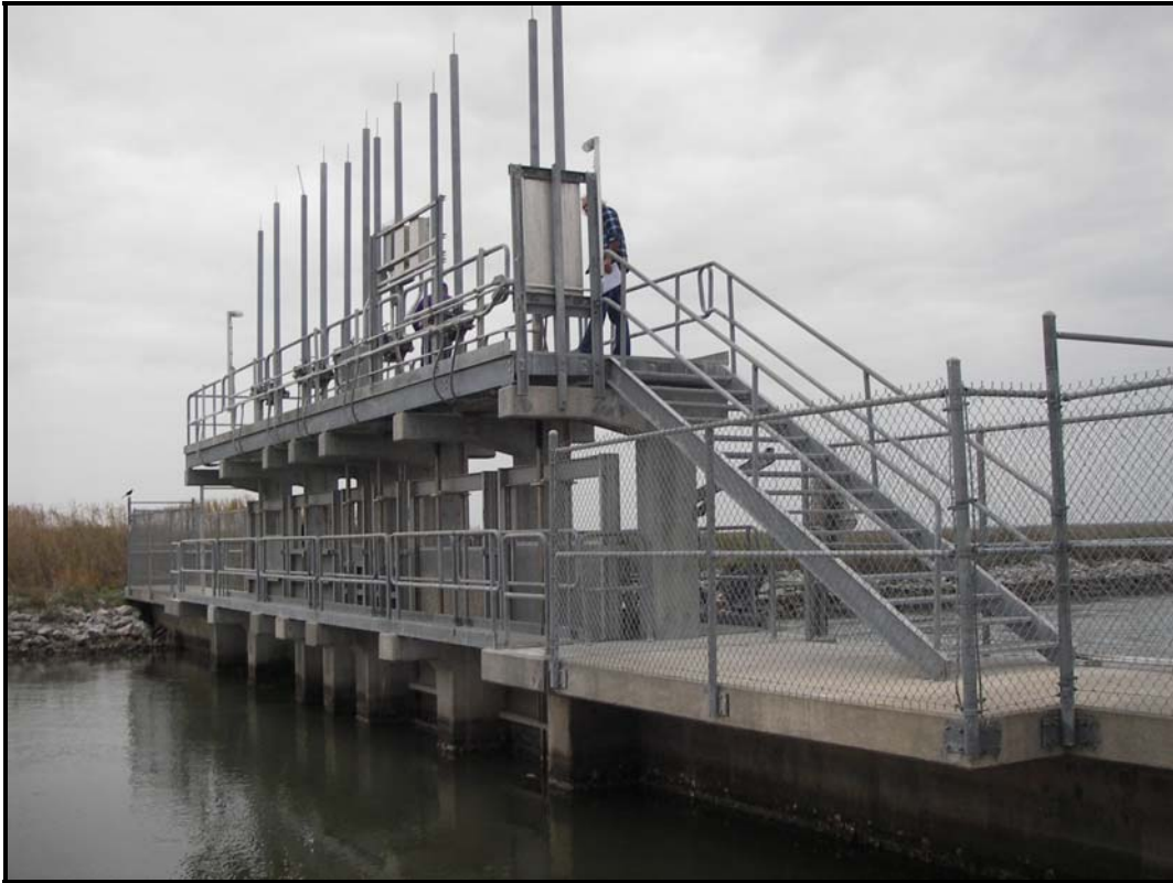
Photo No. 1, Hog Island Gully Structure
