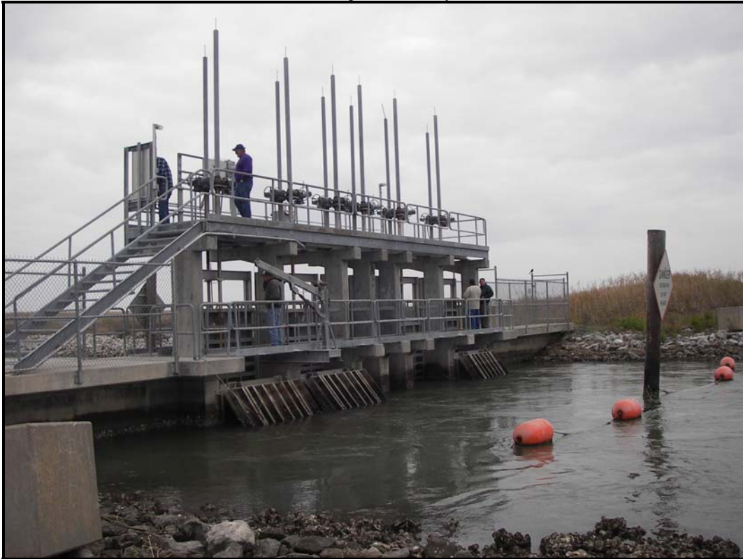
Photo No. 2, Hog Island Gully Structure
