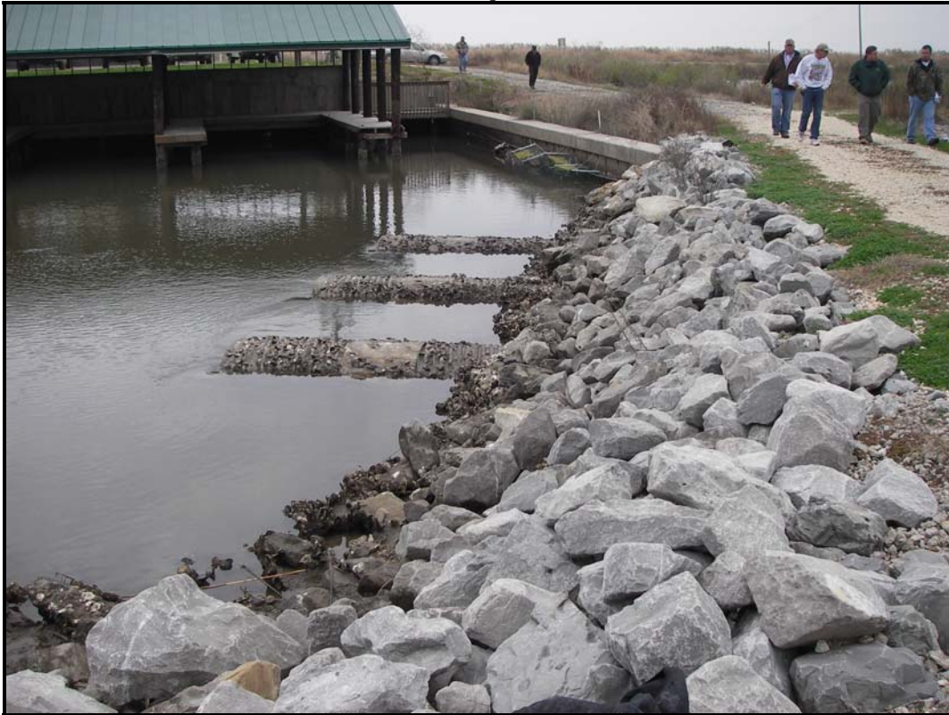
Photo No. 4, Headquarters Structure
