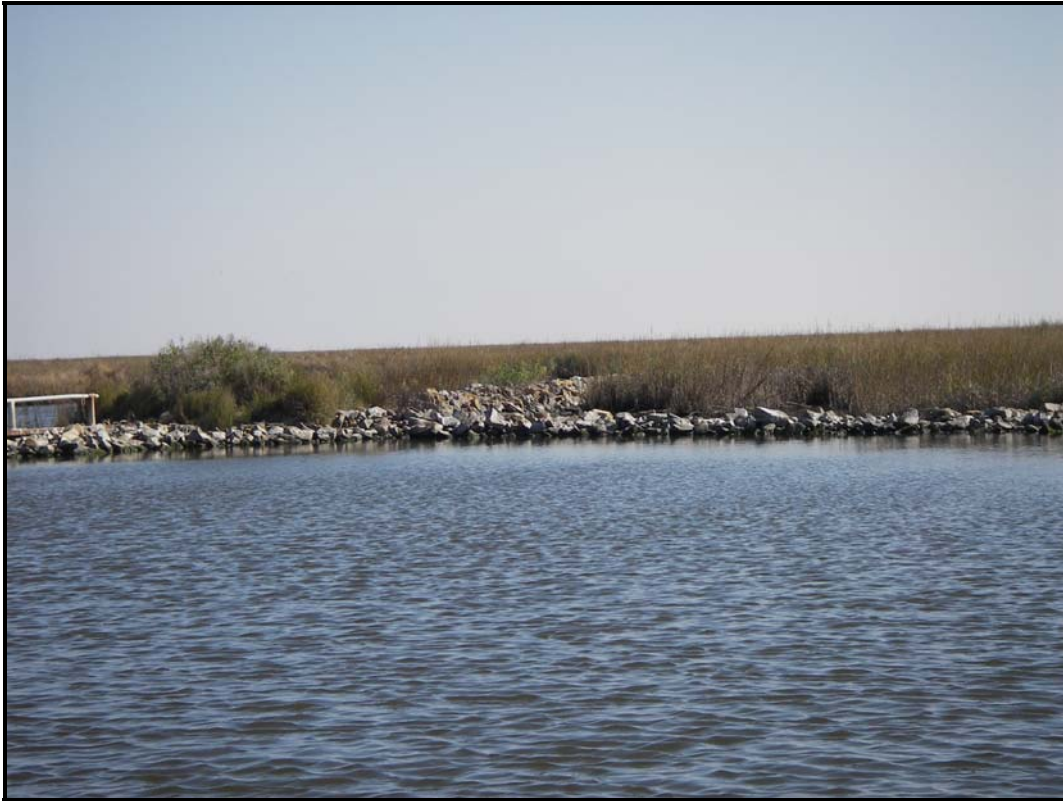
Photo 1 , Grand Bayou Weir, view of rock east side.
