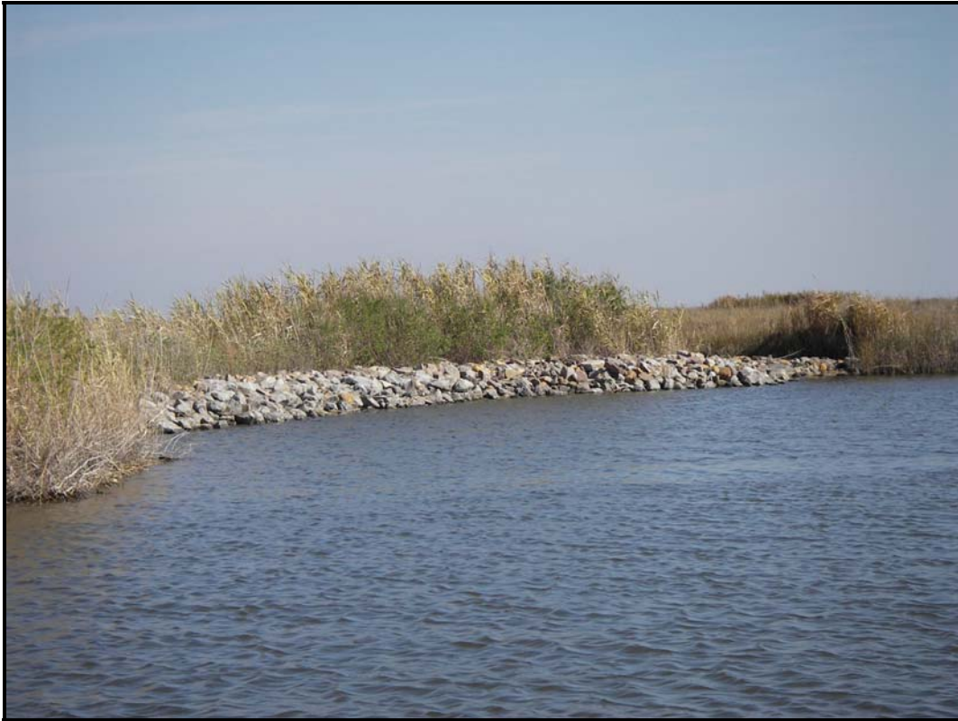
Photo No. 5, Mangrove Weir, view of rock armor east side.
