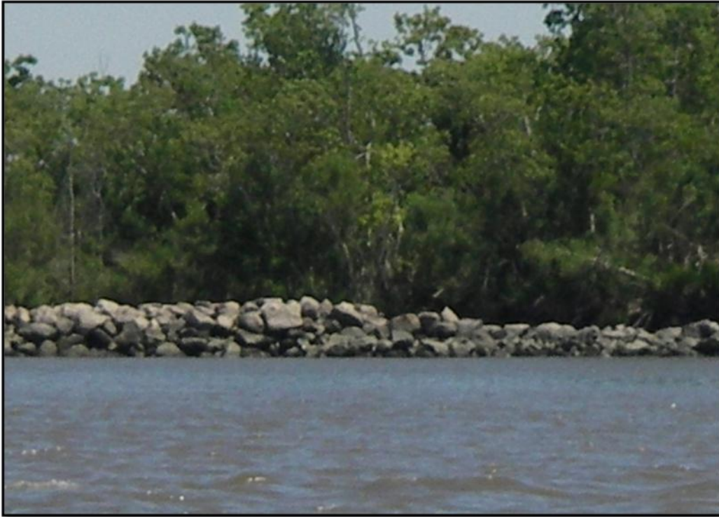
Photo No. 1, Typical rock dike
