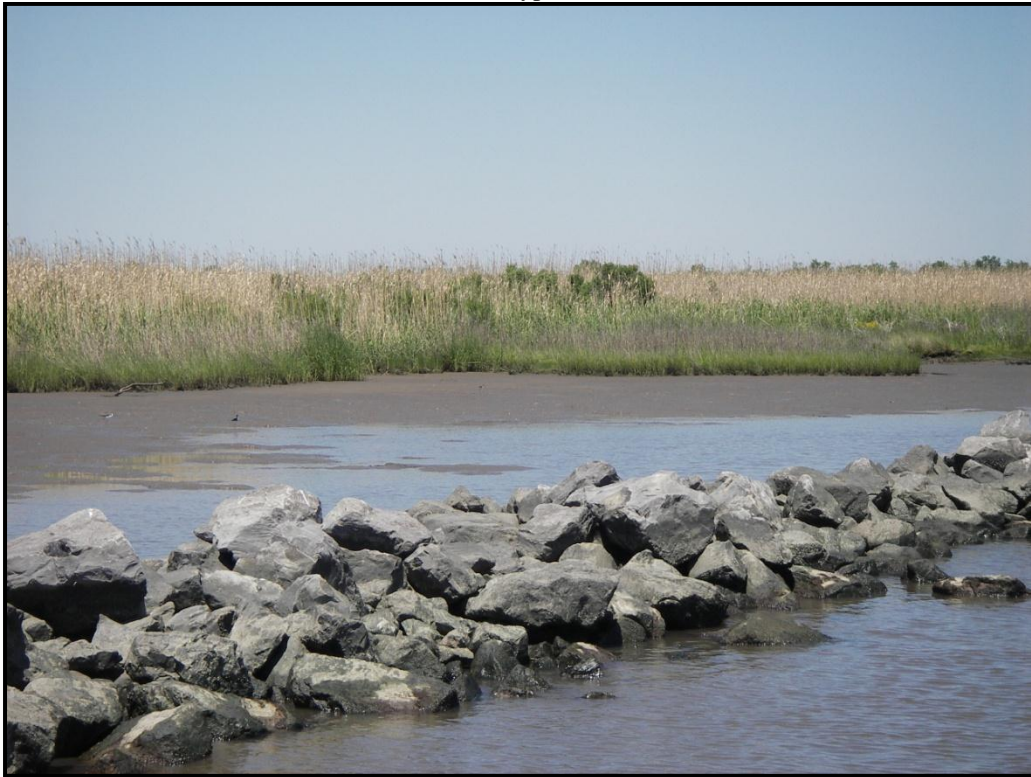
Photo No. 2, View showing accretion behind rock dike
