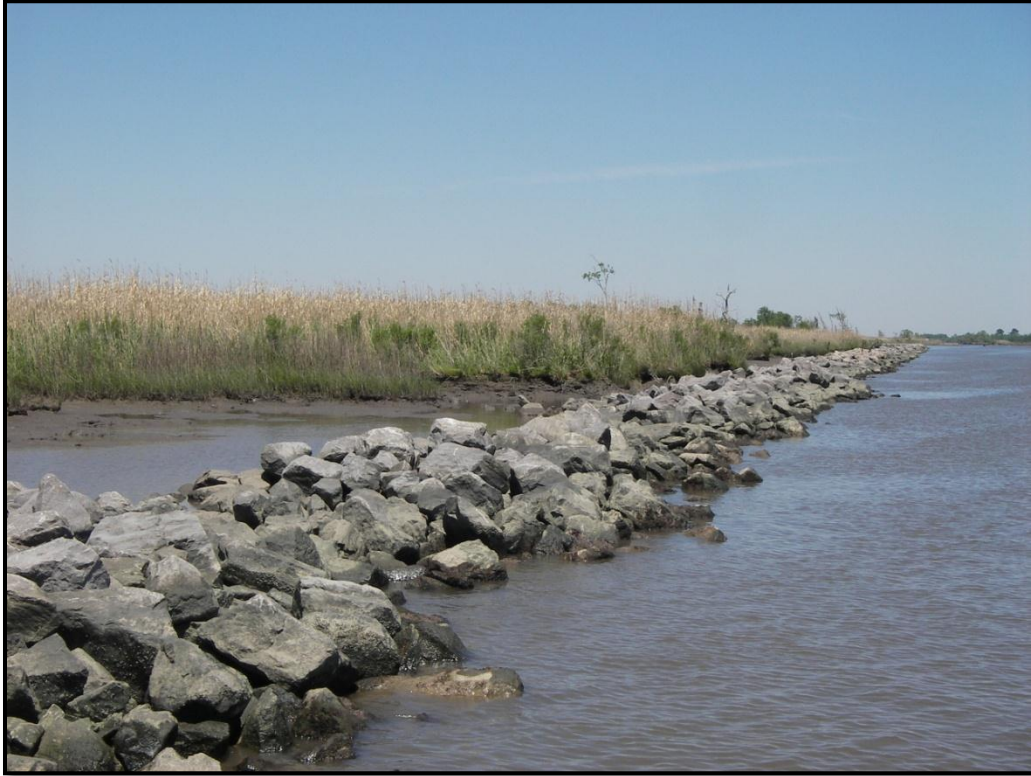
Photo No. 1, Typical rock dike
