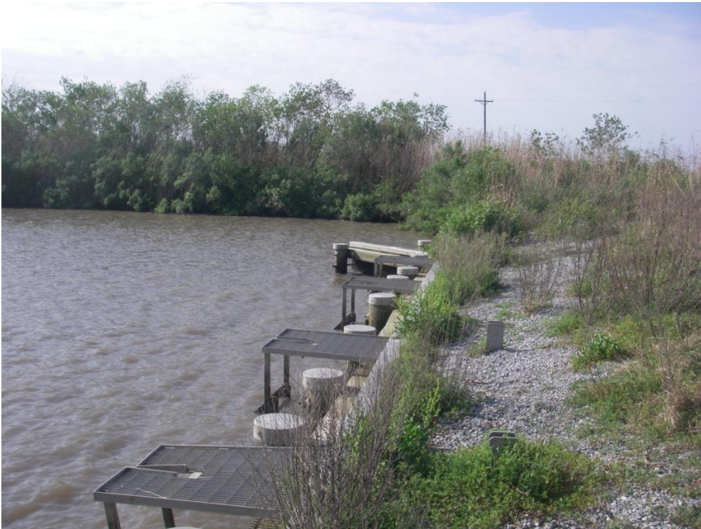
Photo No. 3 , Outlet side of structure
