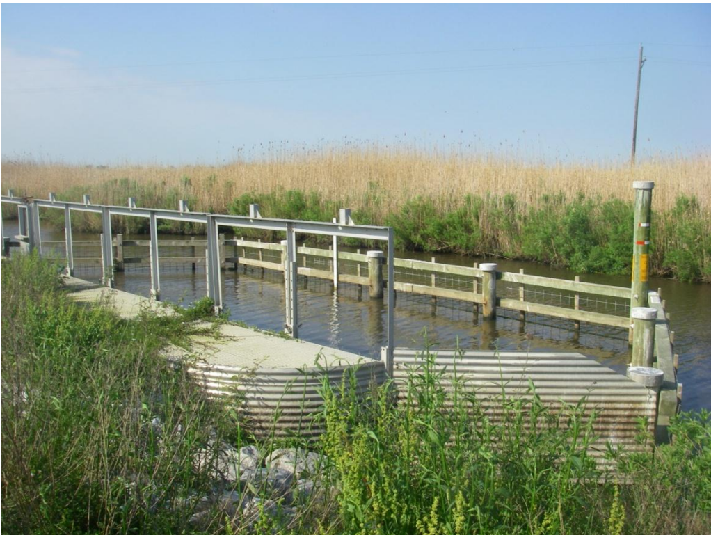
Photo No. 2, Inlet side of structure
