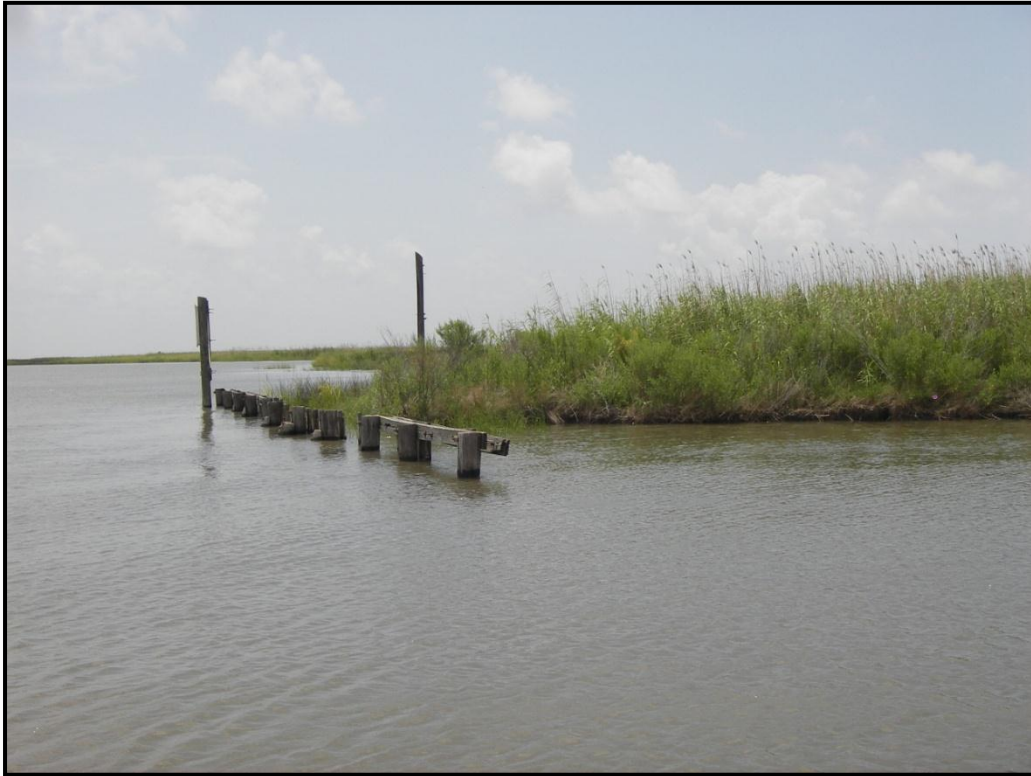
Photo 7, Area 3, near bulkhead on north end.
