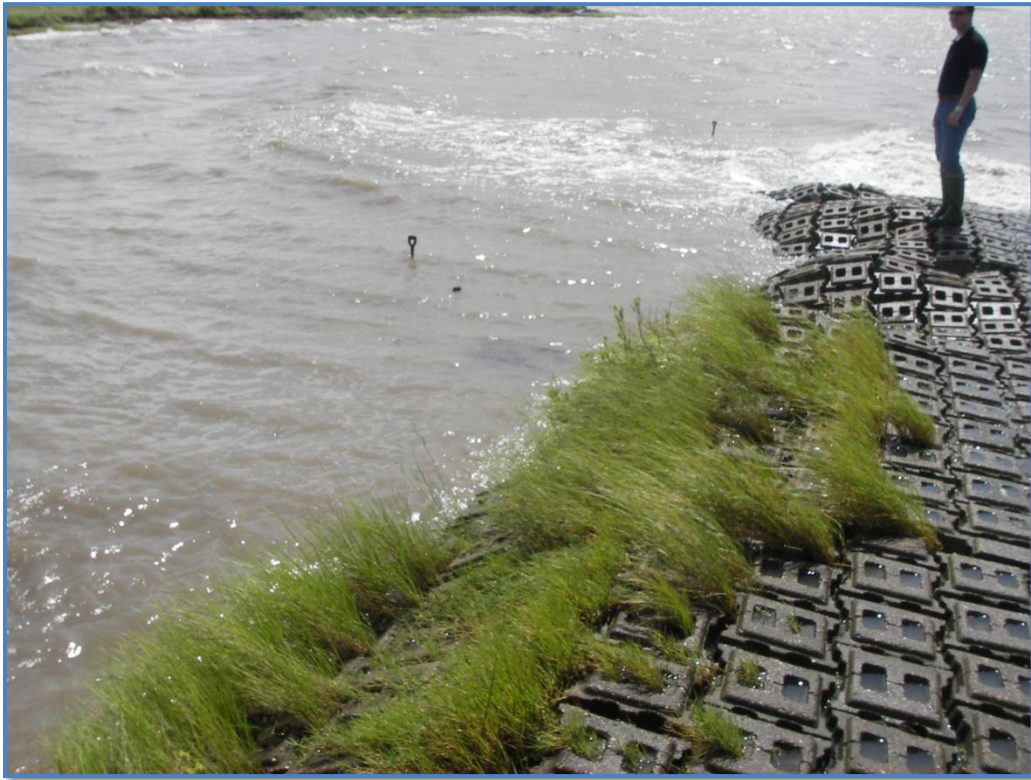
Photo 5, Area 2, East side of concrete mats.
