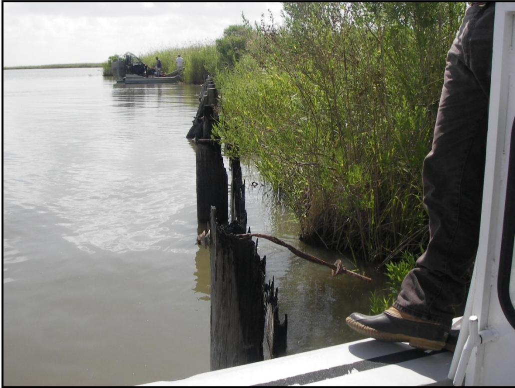
Photo 1, Area 1, Timber bulkhead.
