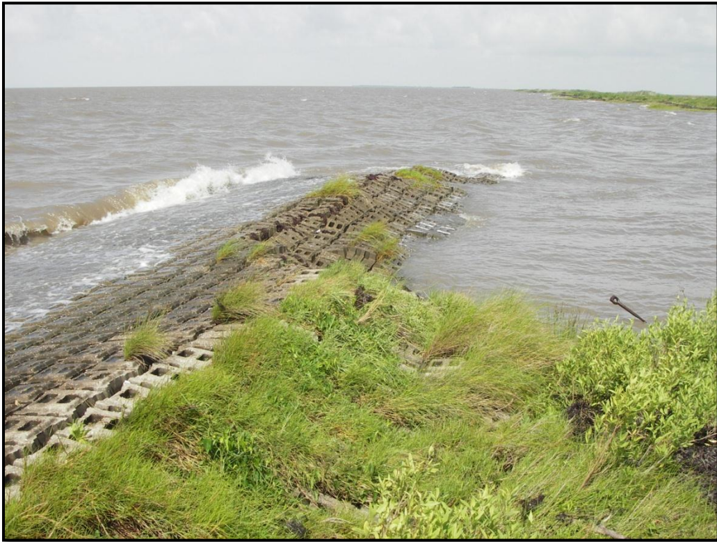
Photo 3, Area 2, West side of concrete mats.
