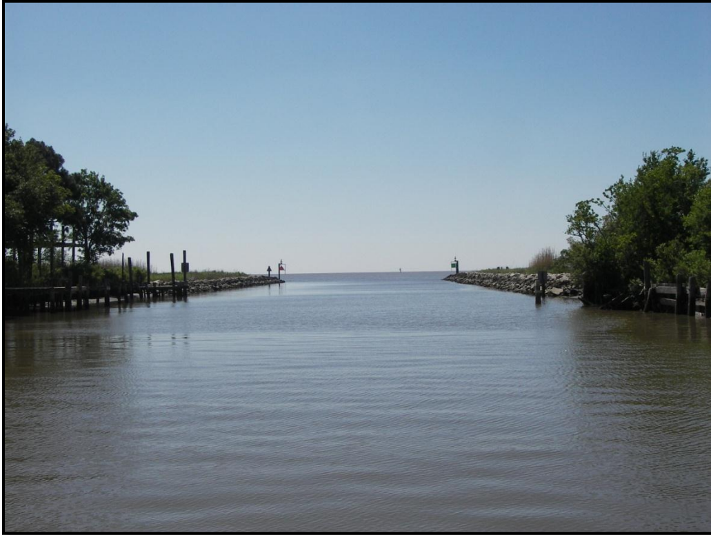
Photo No. 1, View of Boston Canal at the bay shore looking South
