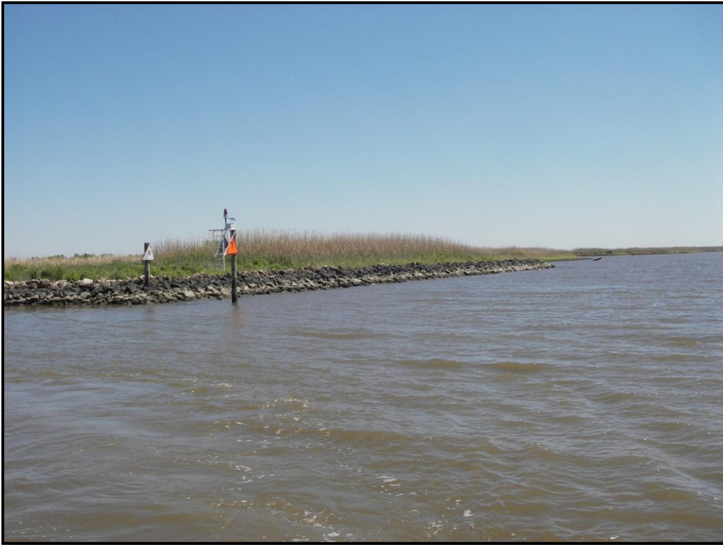
Photo No. 3, View of eastern rock dike
