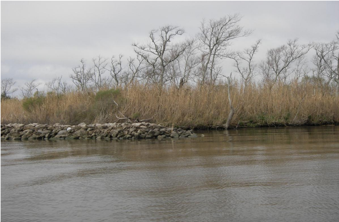
Photo No. 1 —south tie in
