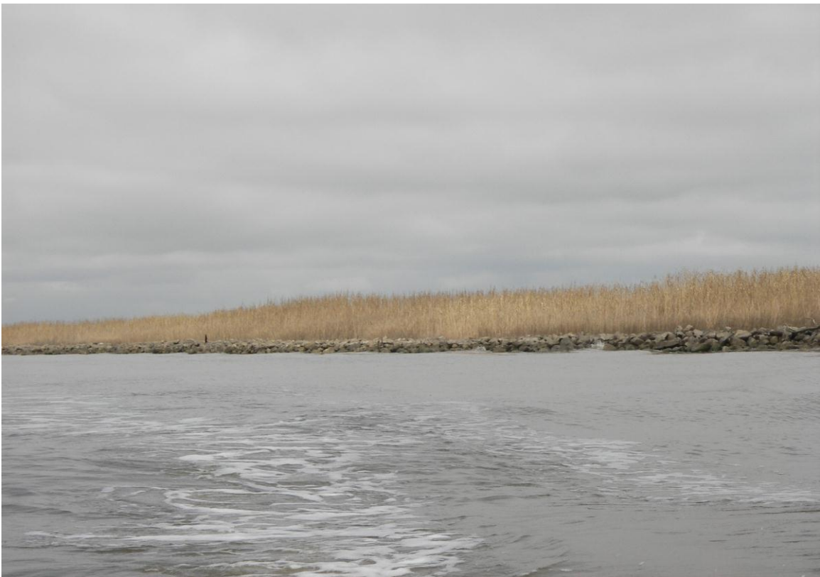
Photo No. 2 —typical section of dike
