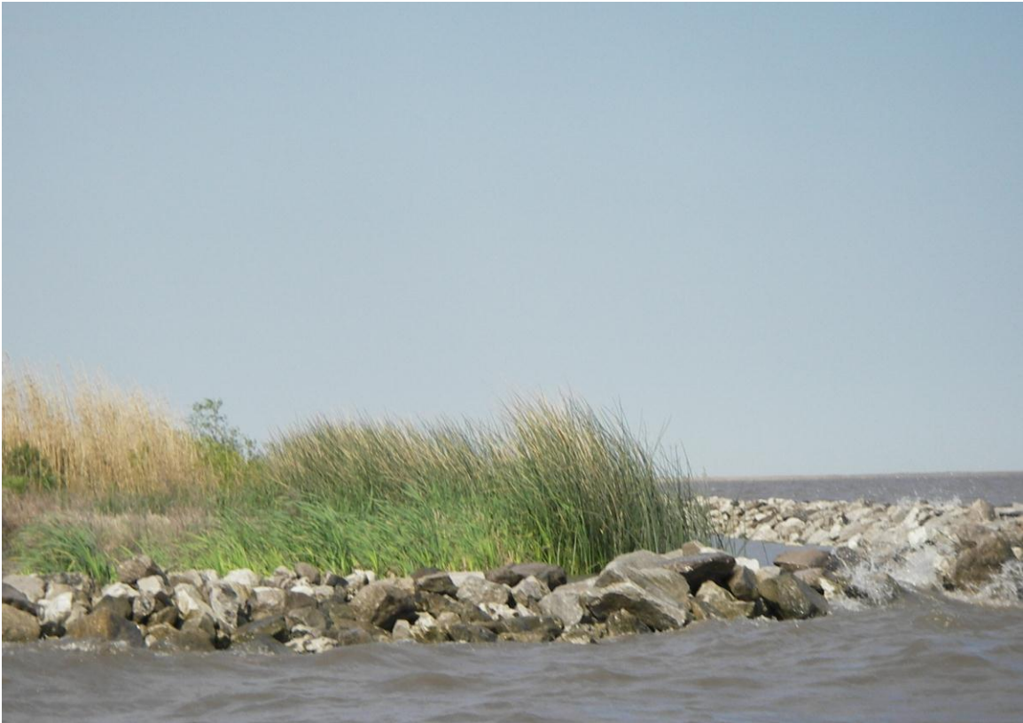
Photo No. 1, typical section of rock dike
