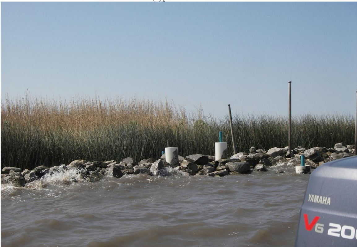
Photo No. 2, test section
