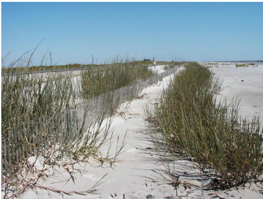
Figure 8b. View of the Sand Fencing and Vegetation Plantings at Station CS31-150 taken in October 2004. The photograph is facing east.
