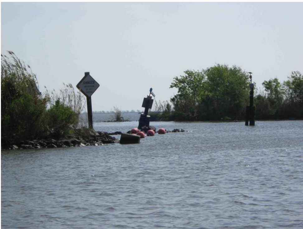
Photo #2 - The Bayou Dupont Canal Weir. Note the leaning piling cluster with the navigation light.
