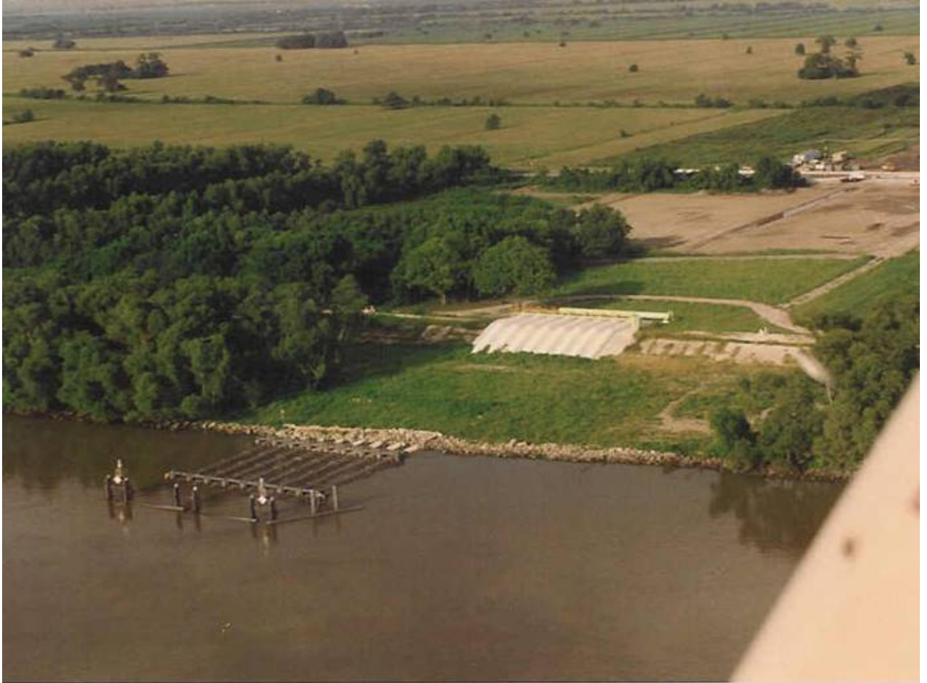
Figure 1. Siphons constructed in 1992 as part of the Naomi-Siphon Diversion (BA-03) project and funded by the state of Louisiana. Mississippi River water is siphoned from the river intakes, discharged into a ponding area, and distributed through a single channel into the surrounding marshes.
