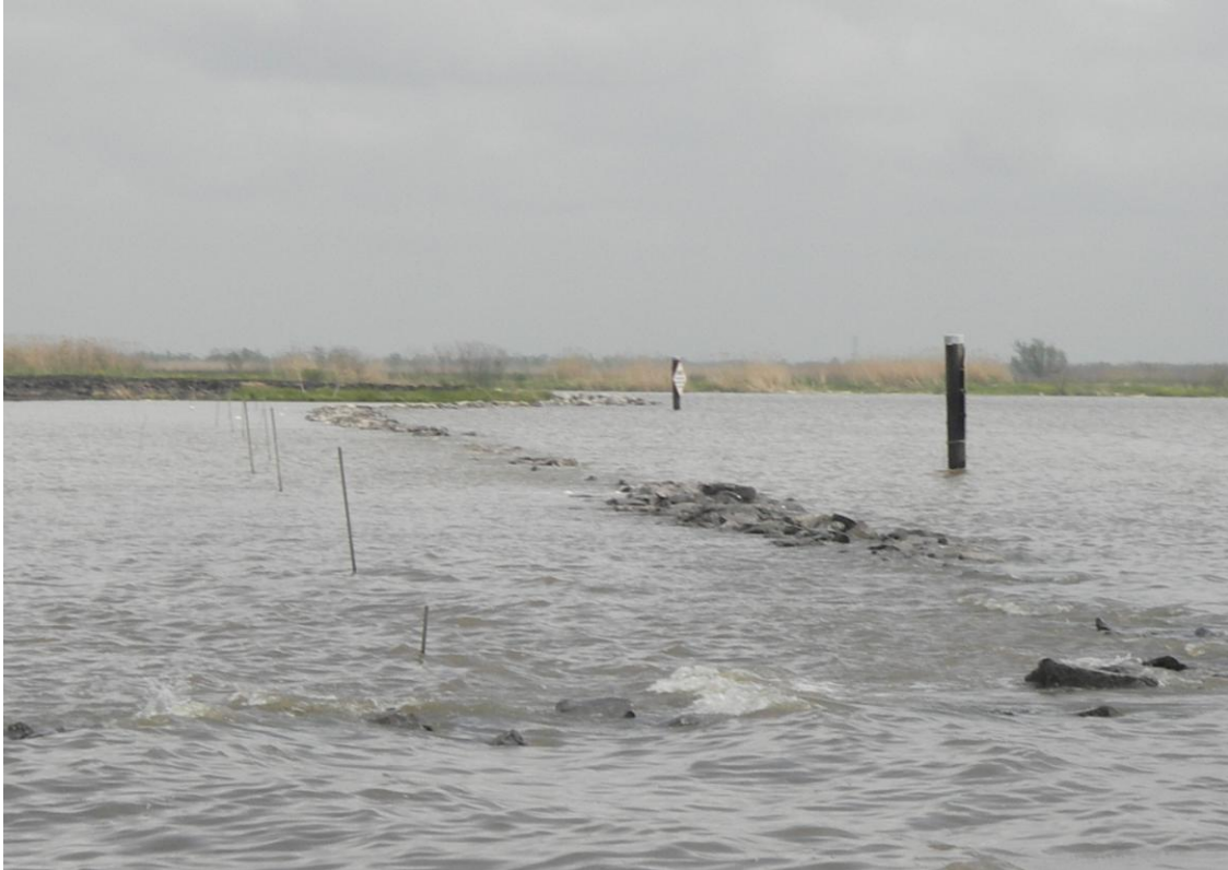
Photo 17 —Typical settled section and signage of School Bus dike
