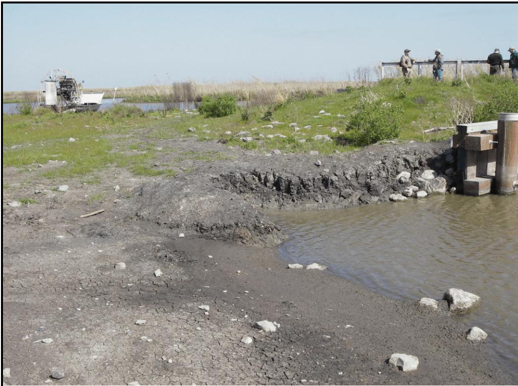
Photo No. 3, View showing minor erosion on SW quadrant of outlet side of New Cop-Cop Structure.
