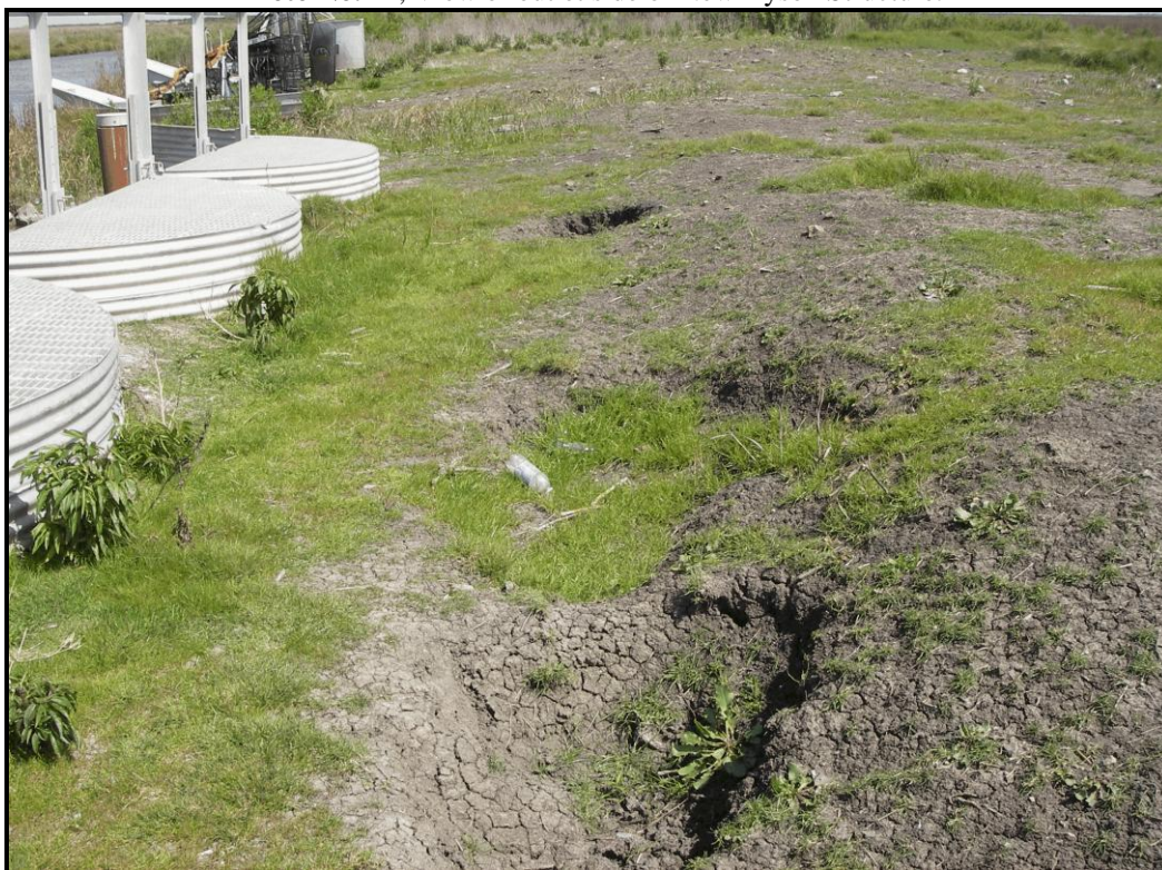
Photo No. 12, View showing three minor settlement areas atop the New Dyson Structure.
