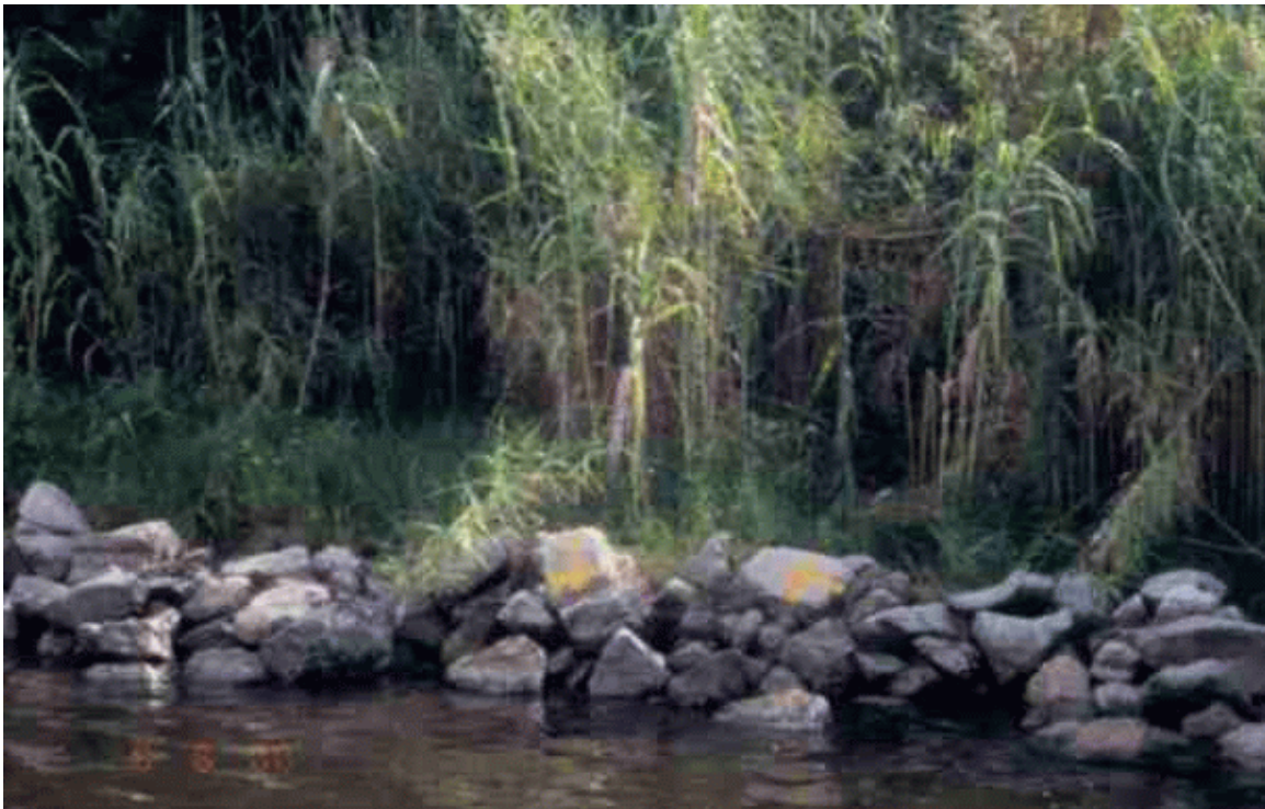
Figure 7. Photograph of the Sabine Refuge Protection (CS-18) project 5 yr following construction in August 2000, showing shoreline advance to the rock breakwater at one of the project stations.
