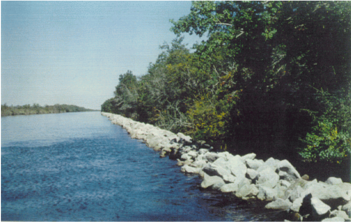
Figure 2. Photograph of the Sabine Refuge Protection (CS-18) project following construction in August 1995, illustrating the shoreline of the impoundment and the installed rock breakwater. Photograph faces north along the eastern bank of the BSC.
