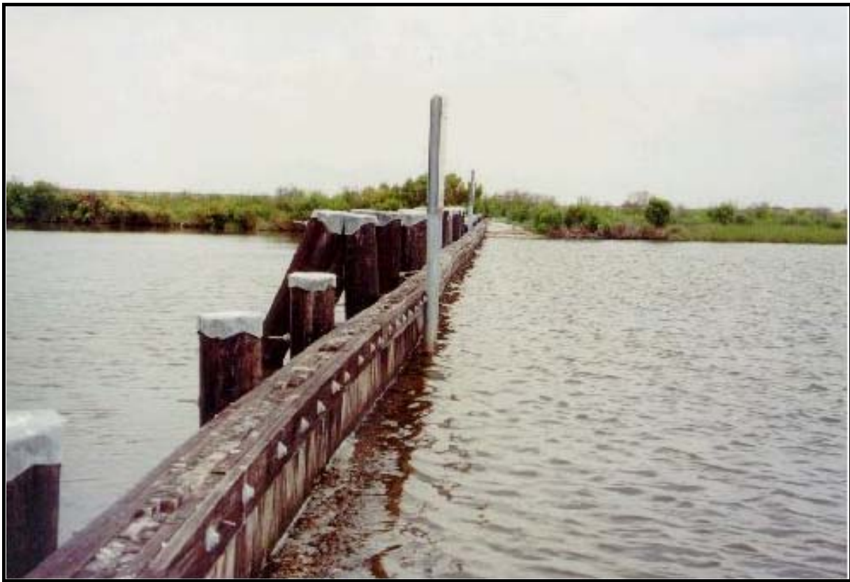
Figure 4. Creosote timber plug. One of seven plugs built by LDNR/CRD within the Phase I project area.
