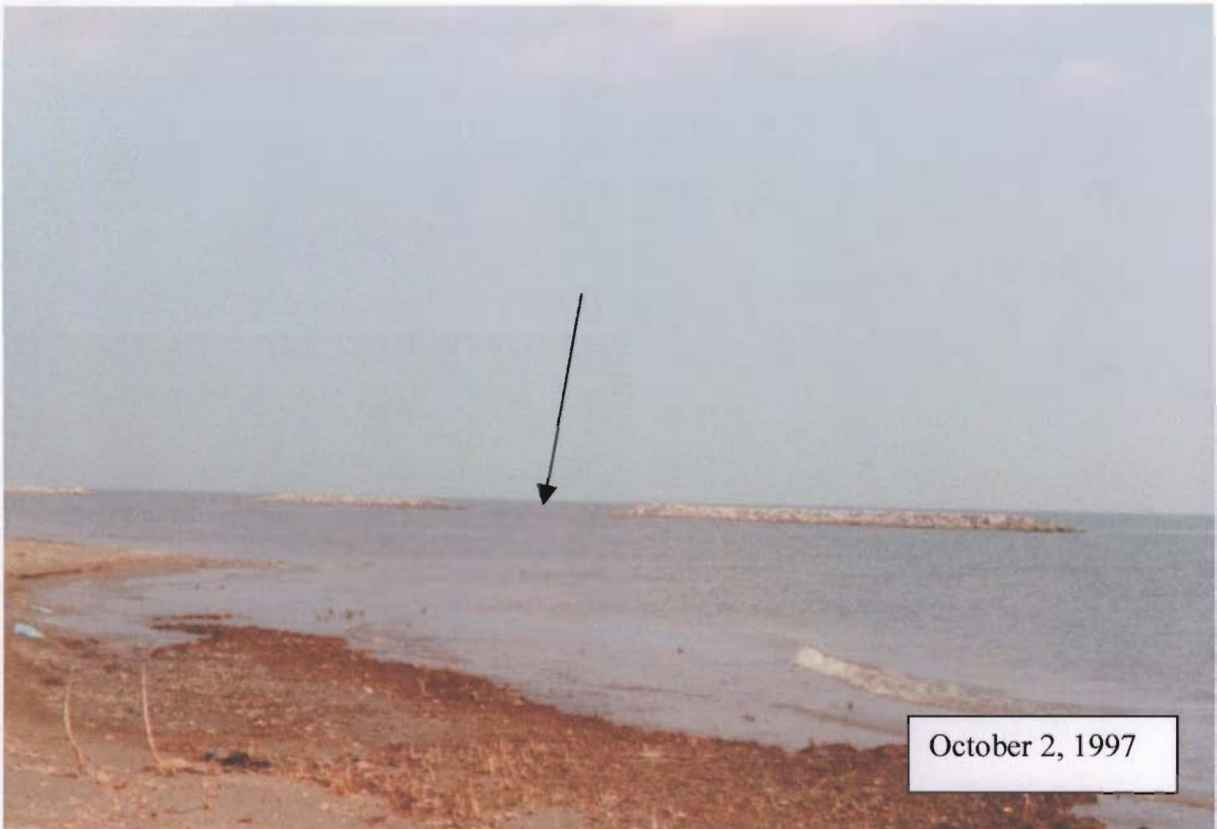
No sand body emerged in the gaps between the breakwaters.
