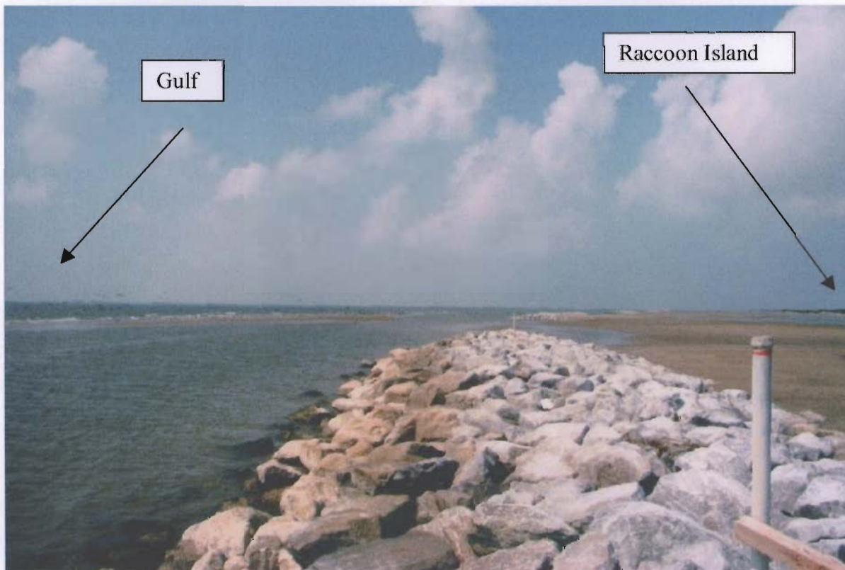
Plate 8. Seaward of the breakwaters, September 1998. Note that the July beach (Plate 6) was eroded. Photograph looking west, September 24, 1998.
