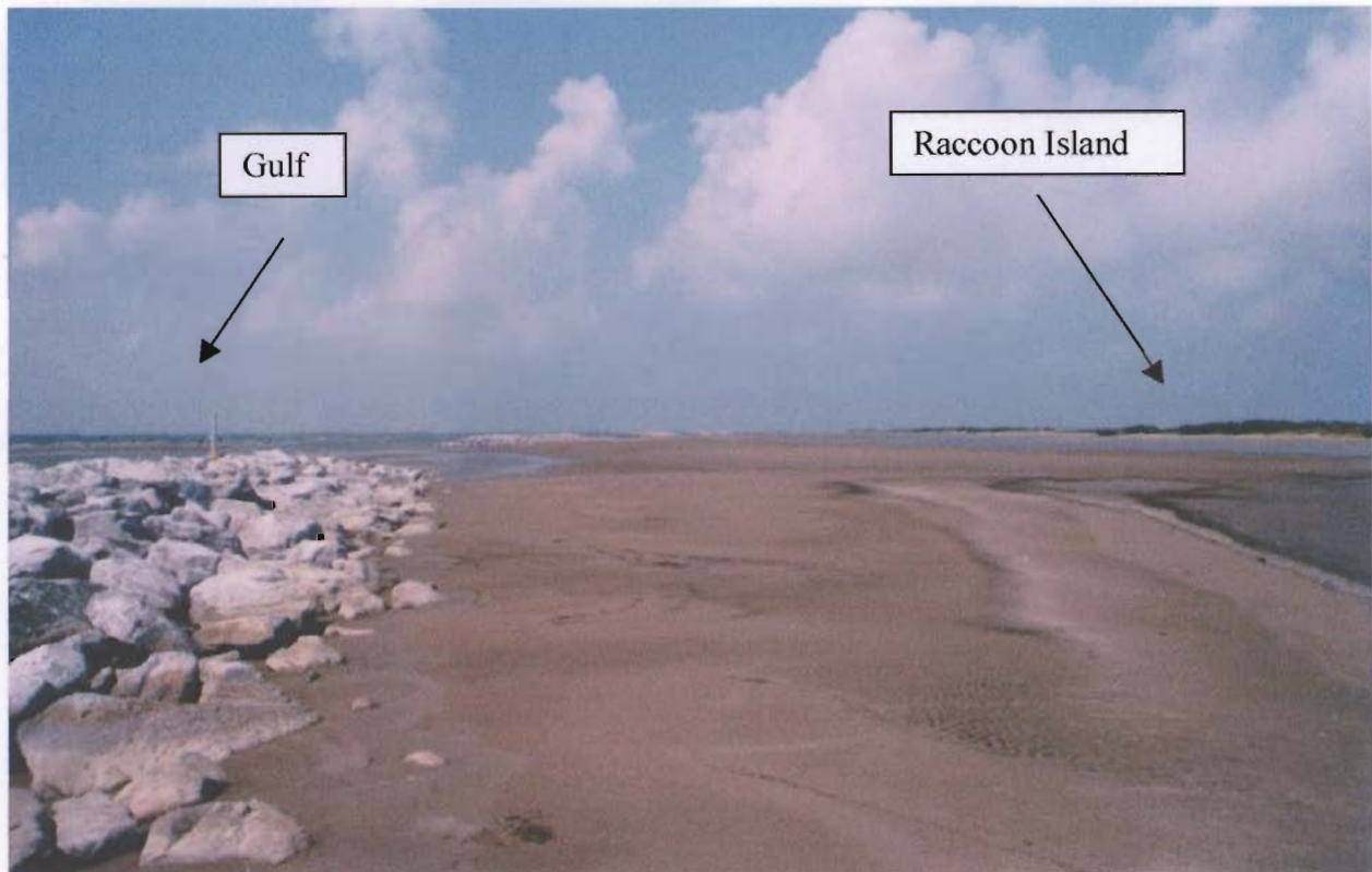
Plate 4. The breakwaters #6, #5, #4, and #3 were connected by an emerged sand body. The sediment that had accumulated immediately seaward of the breakwaters had been eroded between July and September 1998. Note the narrow water body landward of the breakwaters. Photograph looking west, September, 1998.
