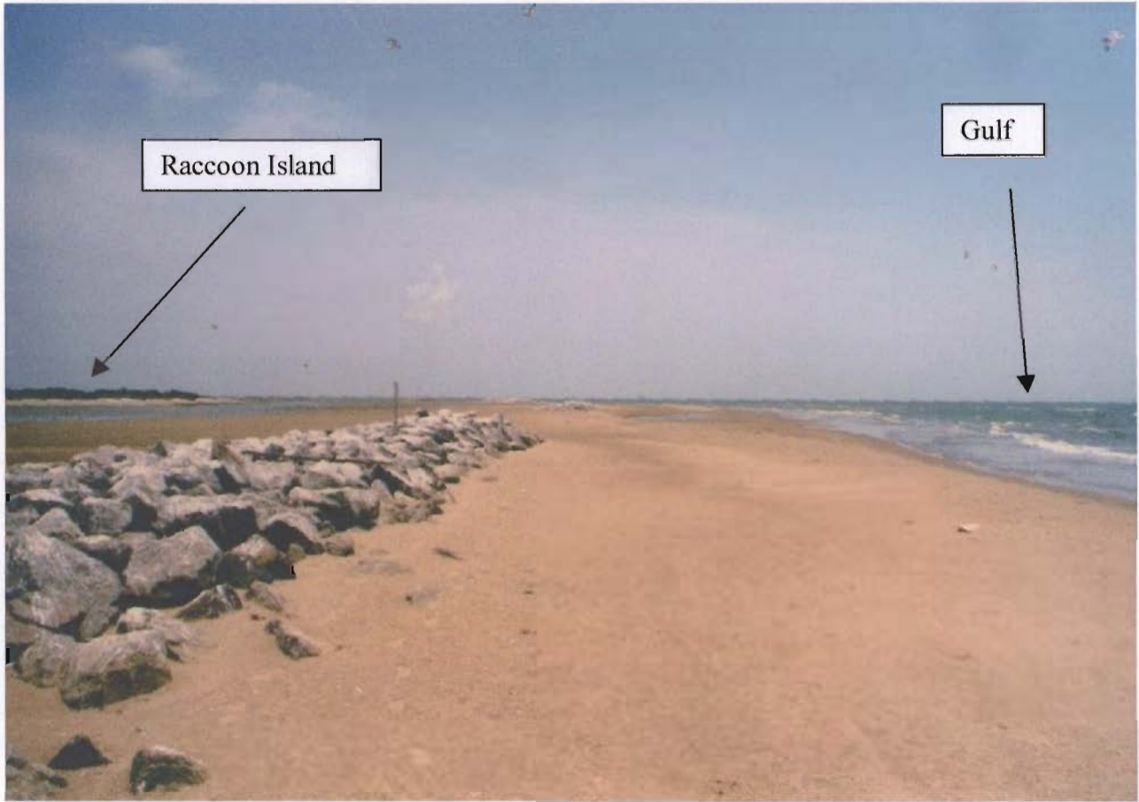
Plate 7. Sand accumulation seaward of the breakwaters, July 31, 1998. Photograph was taken looking east.
