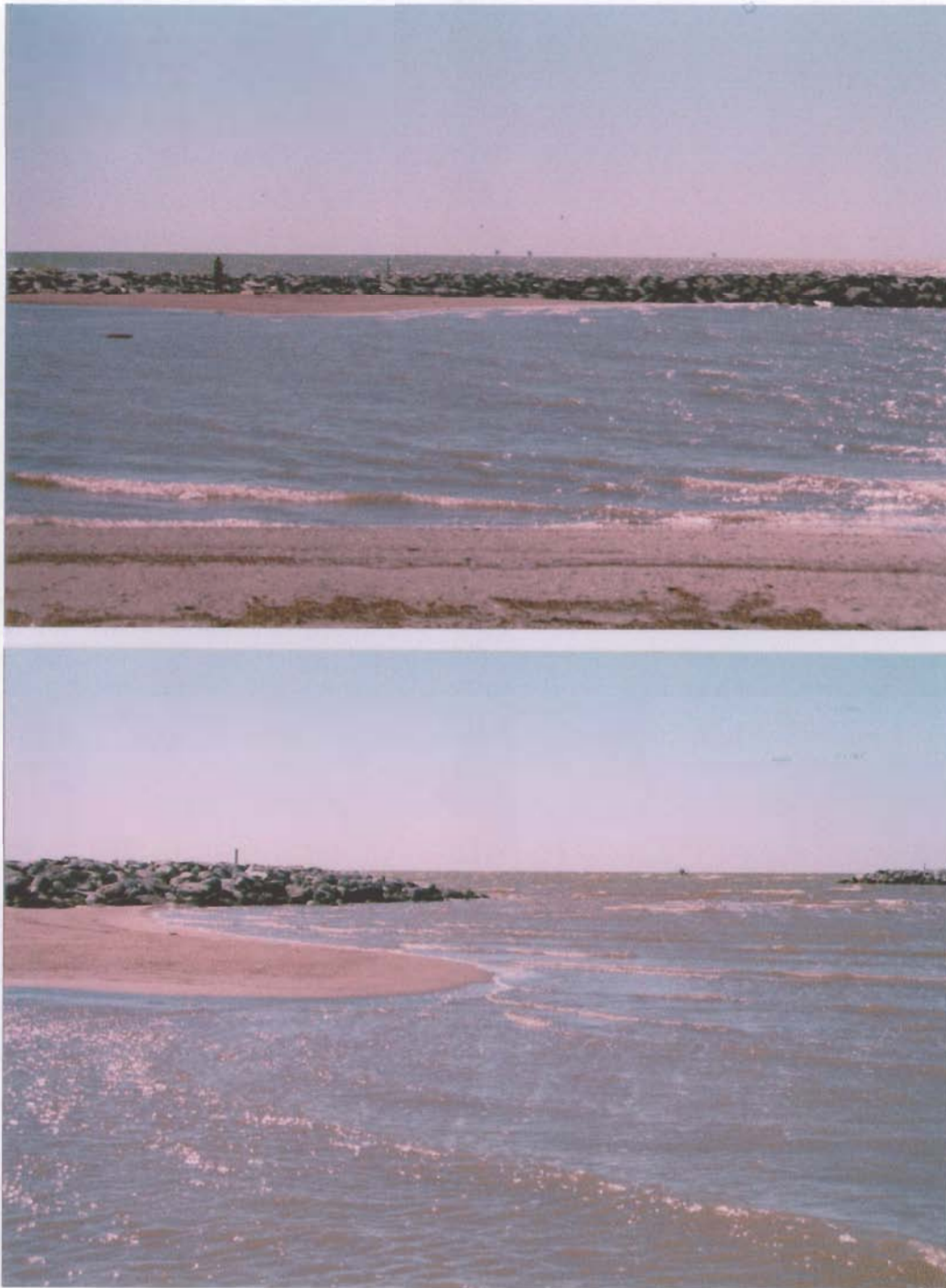
Plate 2. Obliquely incident waves. Upper: oblique waves breaking at the shoreline, looking south from Raccoon Island. Lower: oblique waves propagating through the gap and breaking at the upwind side of the emerged sand body directly behind breakwater #6, looking west from the emerged sand body directly landward of the breakwaters.
