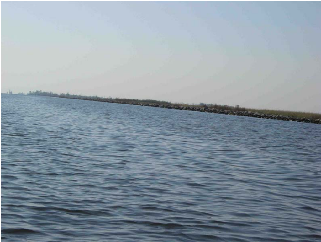
Photo #1 – Shoreline Protection Looking North
