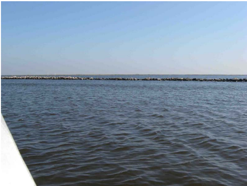
Photo # 2 – Small gap in Shoreline Protection.
