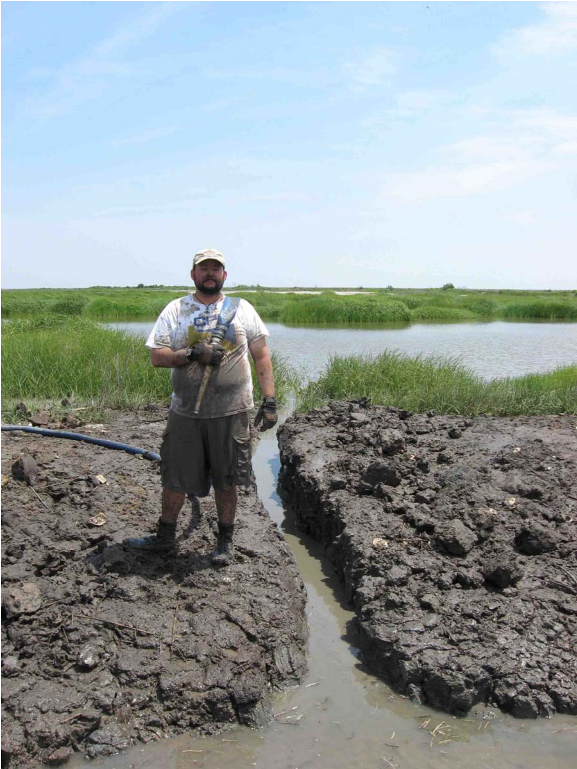
Photo #2 – Hydraulic Dike Gapping.
