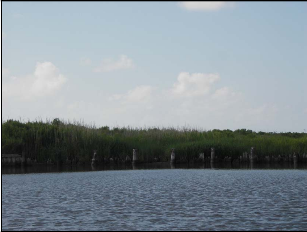
Photo 1, Area 1, View looking south at timber bulkhead.
