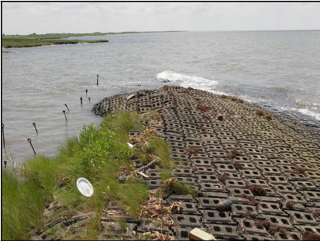
Photo 4, Area 2, East side of concrete mats.
