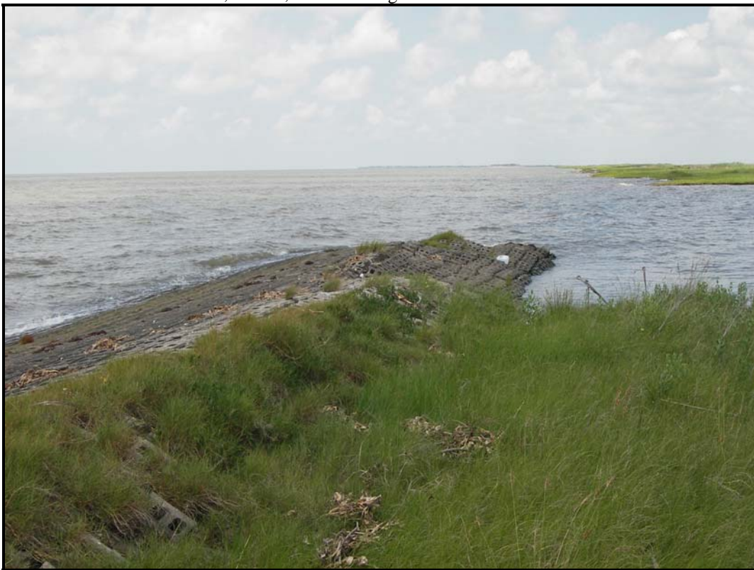
Photo 2, Area 2, West side of concrete mats.
