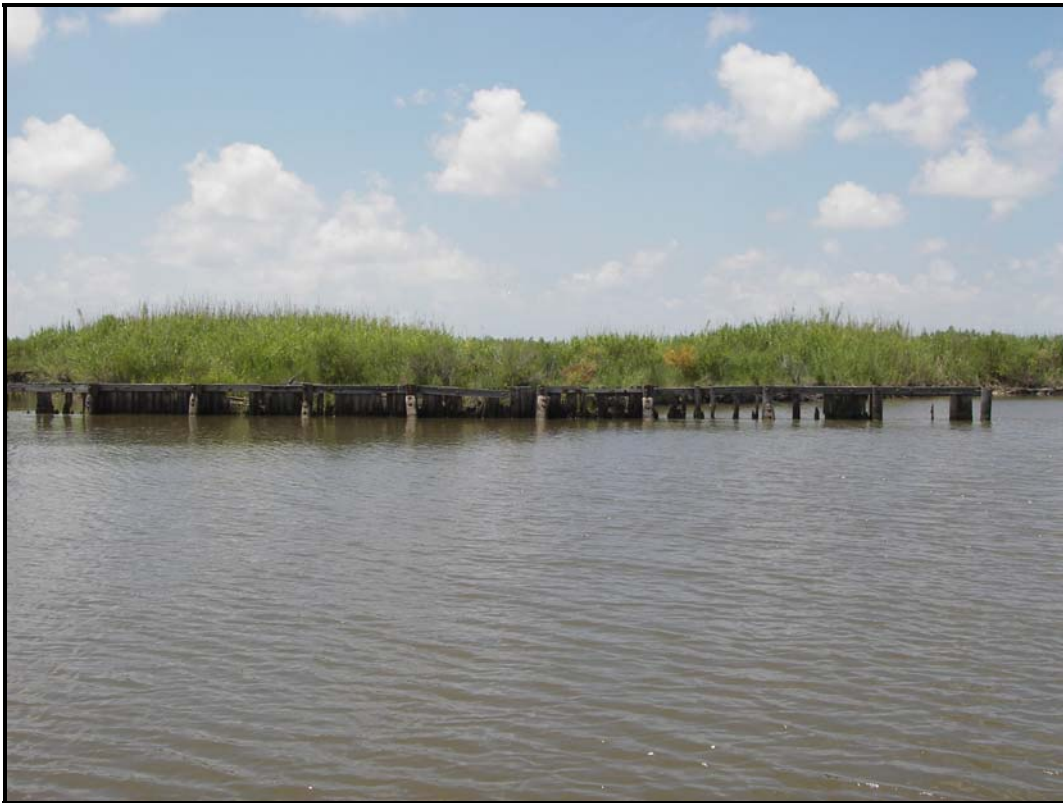
Photo 6, Area 3, near bulkhead on north end.
