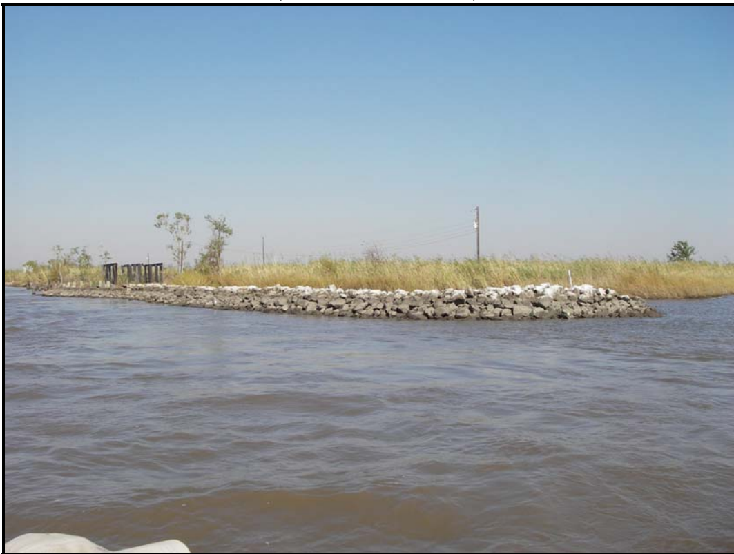
Photo No. 2 , Rock dike at Oaks Canal, east side
