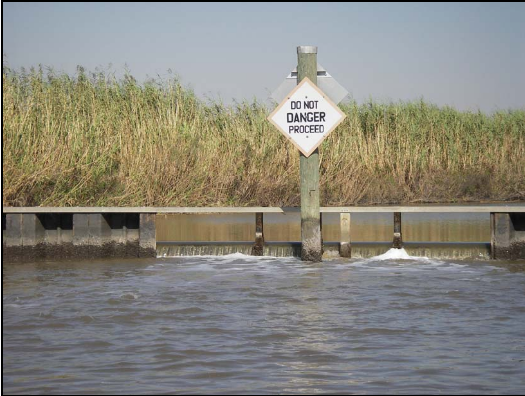
Photo No. 3, Cow Path Structure
