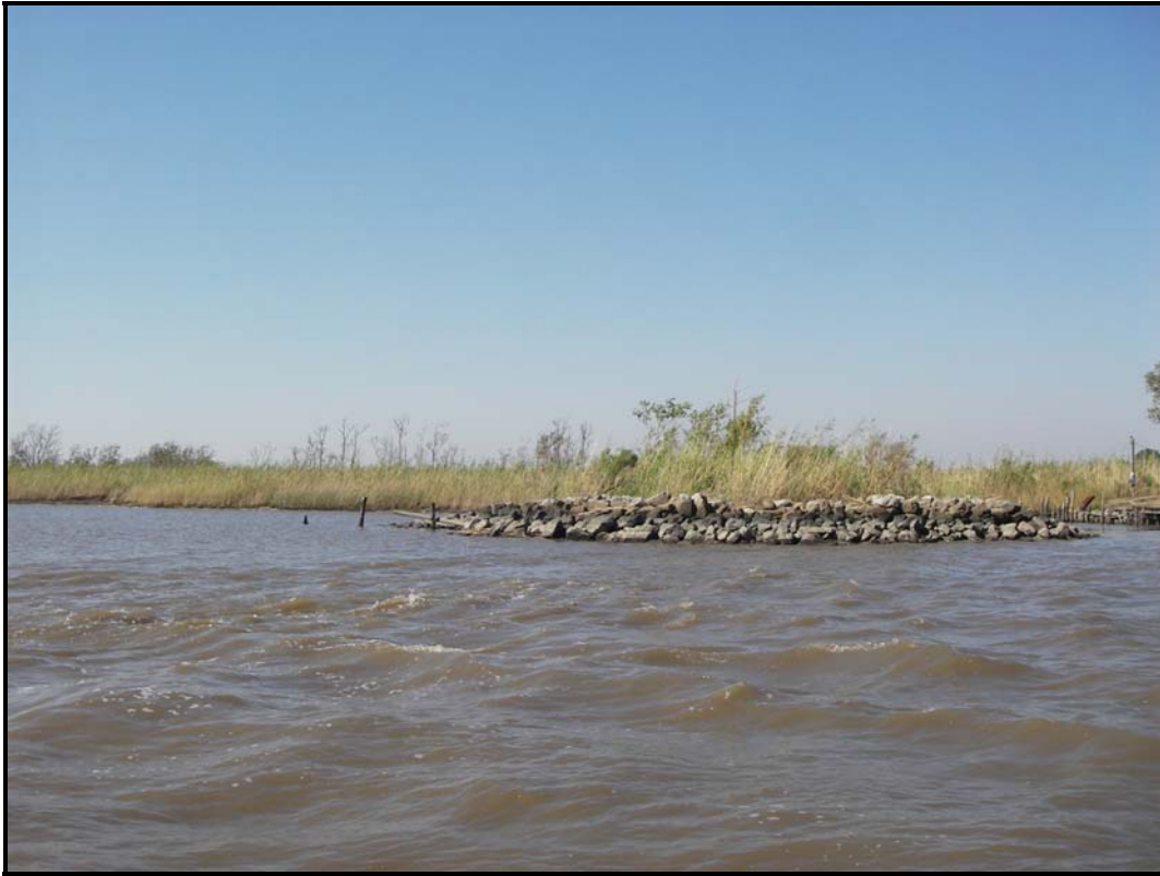
Photo No.1 , Rock dike at Oaks Canal, west side
