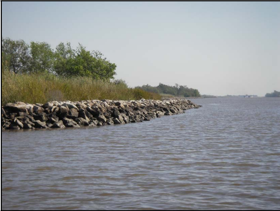
Photo No. 5, Rock along north bank of GIWW
