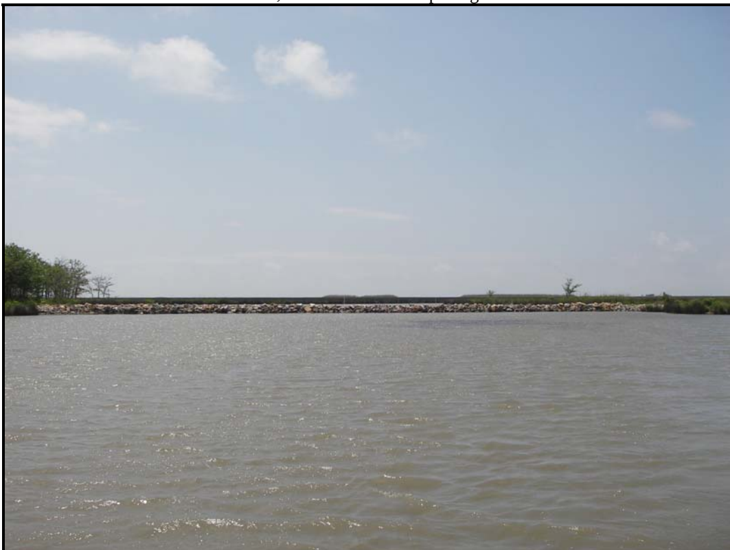
Photo No.2 , Closure No. 1 looking south
