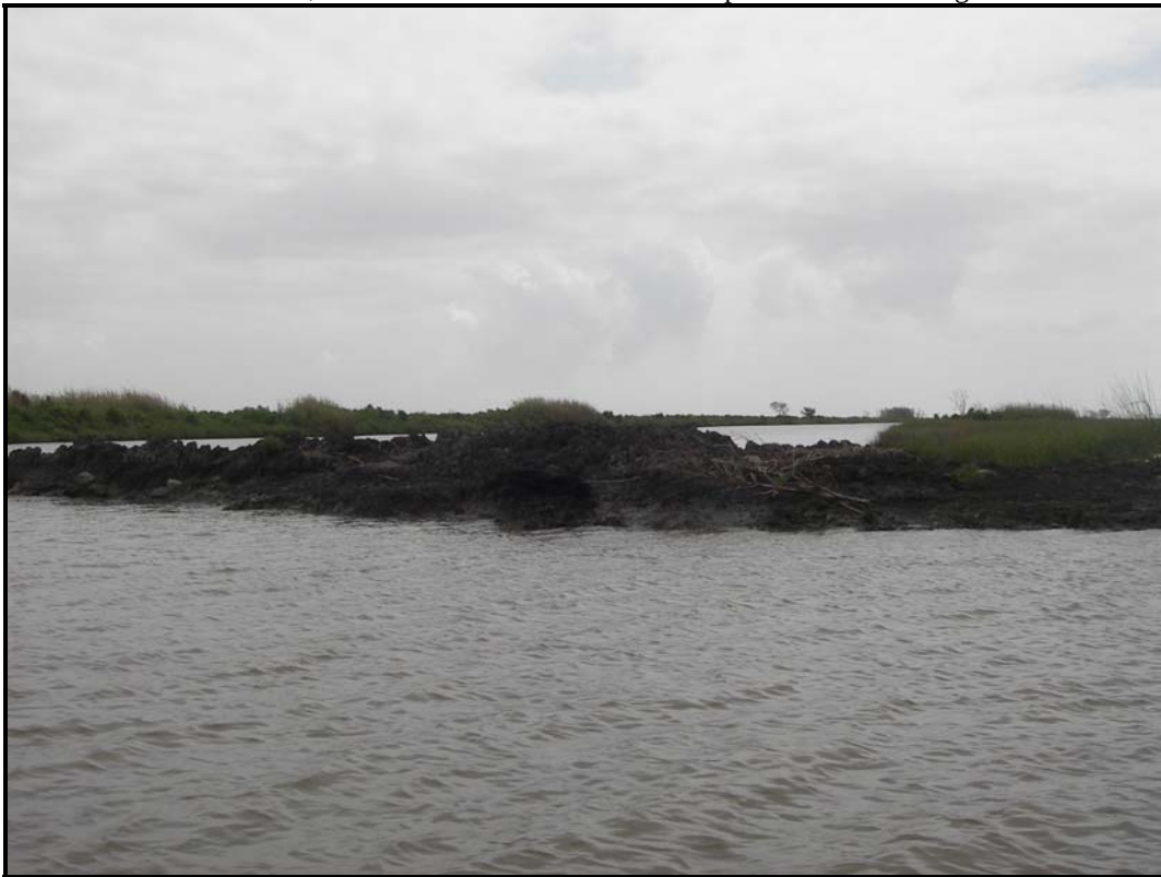
Photo No. 20, Closure No. 8 breach repair with spoil material
