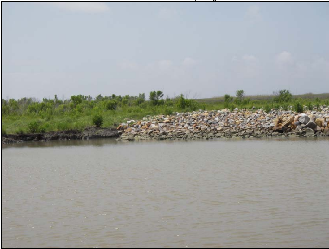
Photo No. 4, Closure No. 2 bank paving east side
