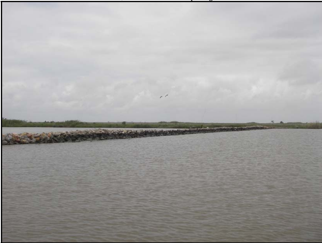
Photo No. 14, Closure No. 6 looking west
