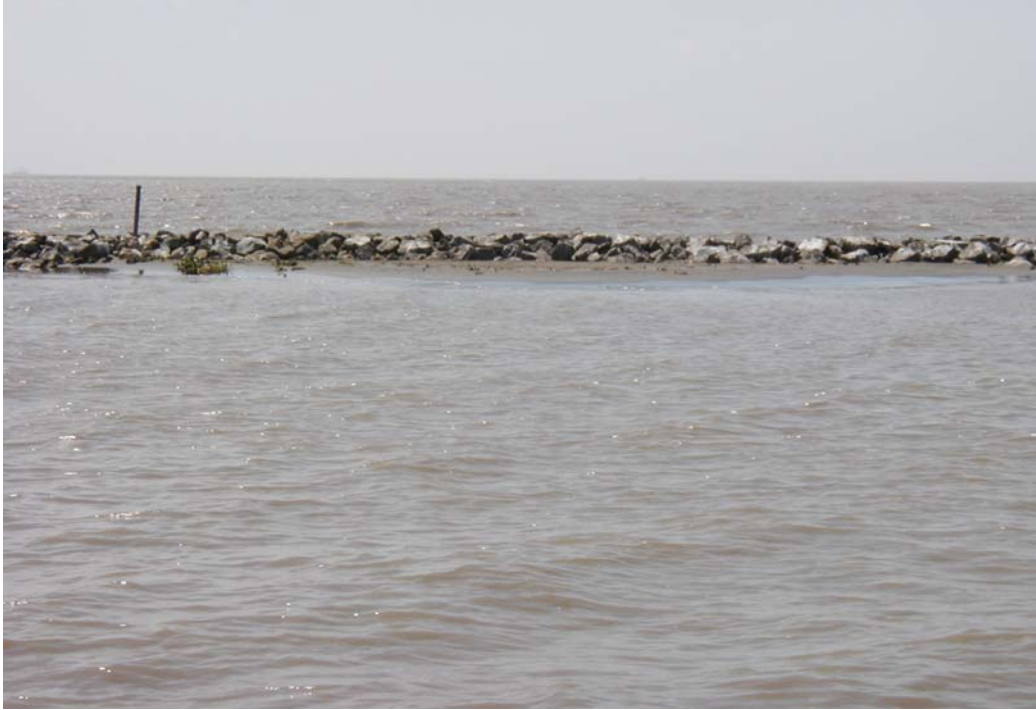
Figure 5. Segmented rock breakwater in project TV-16 area, showing foreshore accreted sand approximately 6 months following construction.
