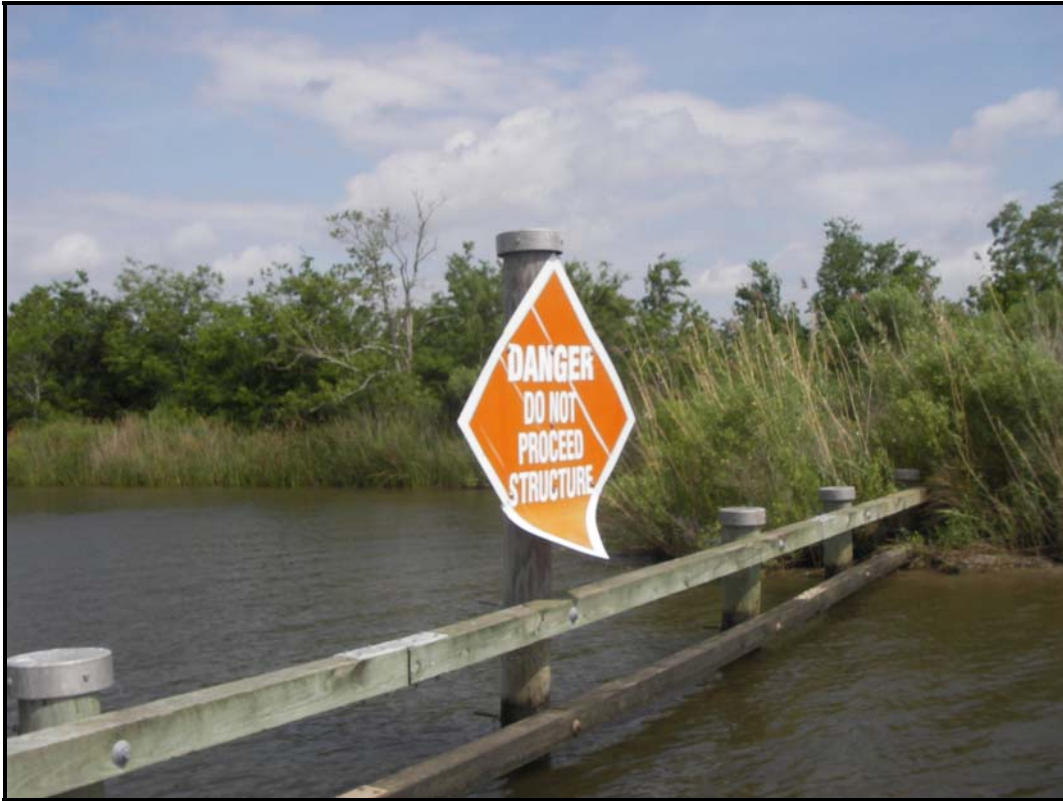
Photo 1 , Marine barrier with signage.
