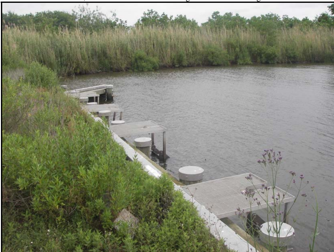
Photo 4 , Outlet side of structure.
